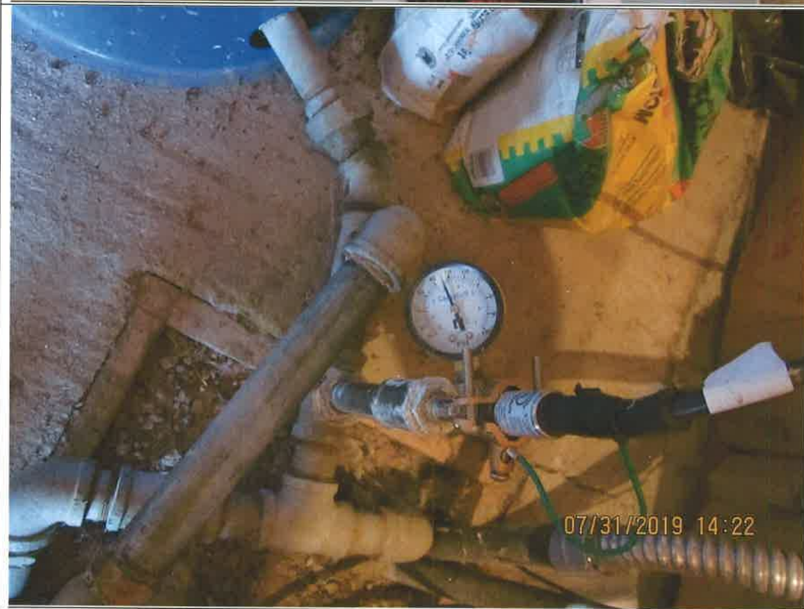
Figure 4. Pressure gage with analog gage showing about 46 psi.
