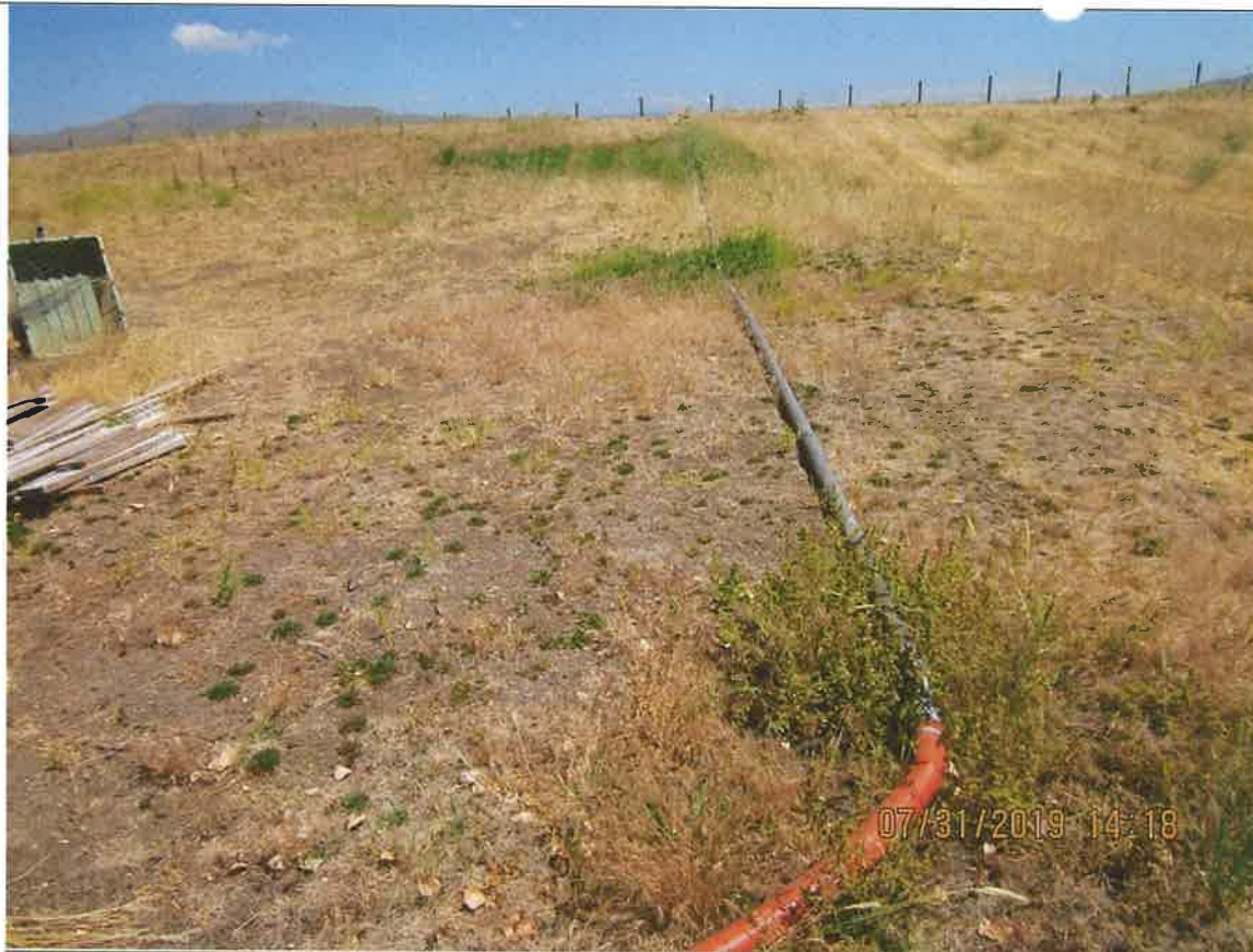
Figure 5. Mainline running uphill from well.
