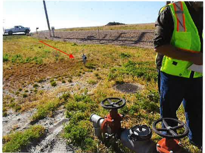
Arrow points to valve for adjacent property field.
