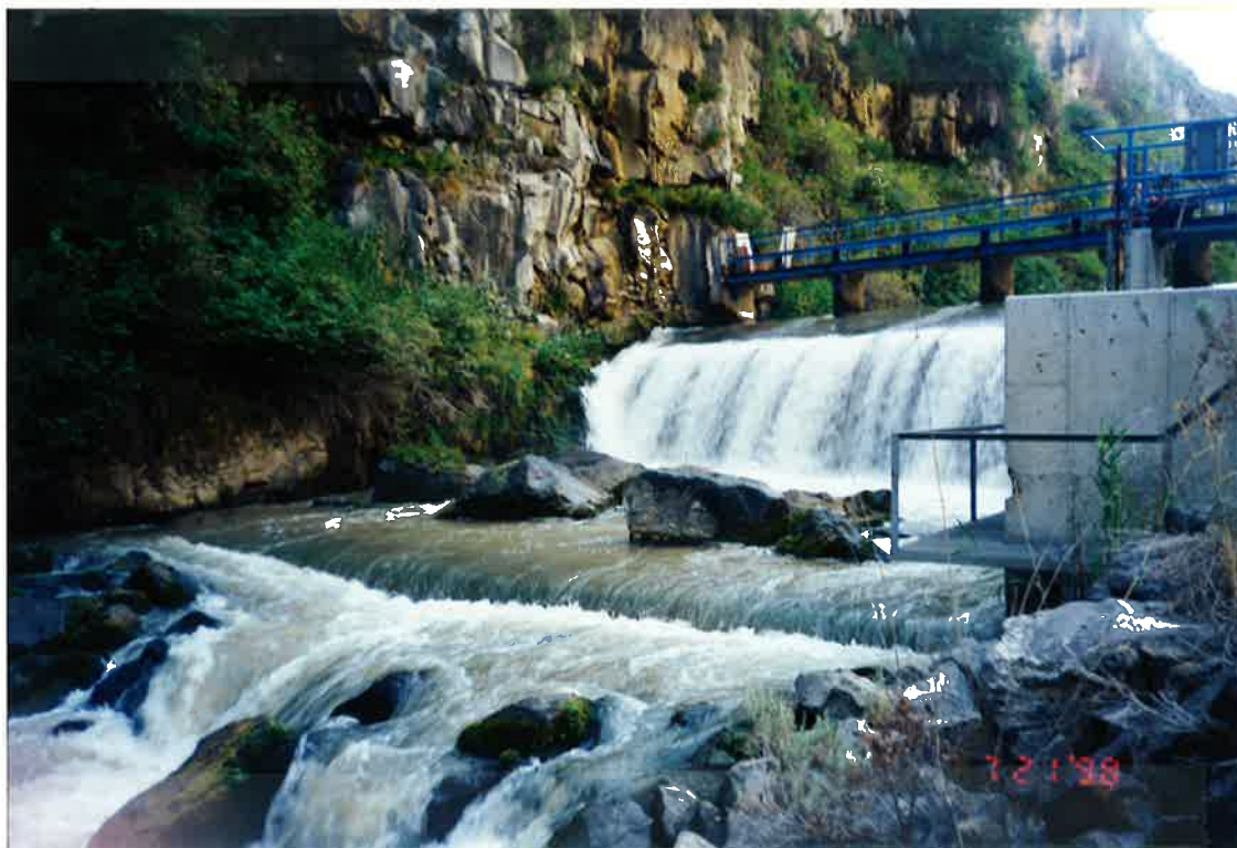
Diverting Works Looking Upstream
