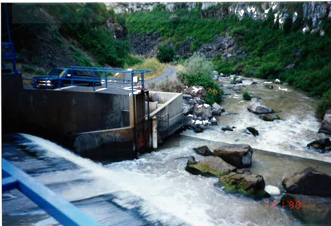
Head of Pipeline Looking Downstream from POD
