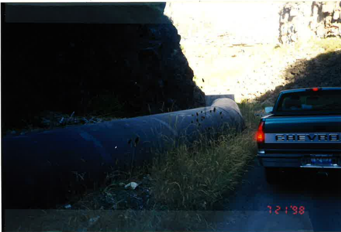
Pipeline From POD To Power Plant
