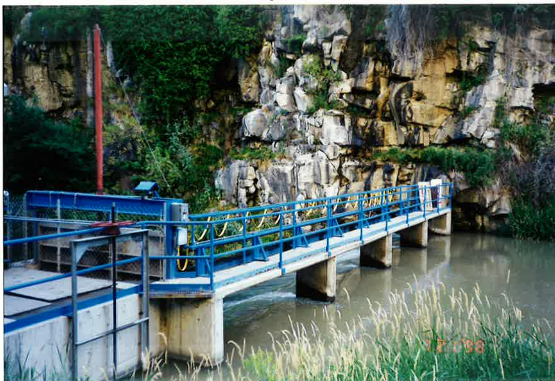
Diverting Works Looking East Across Rock Cr.
