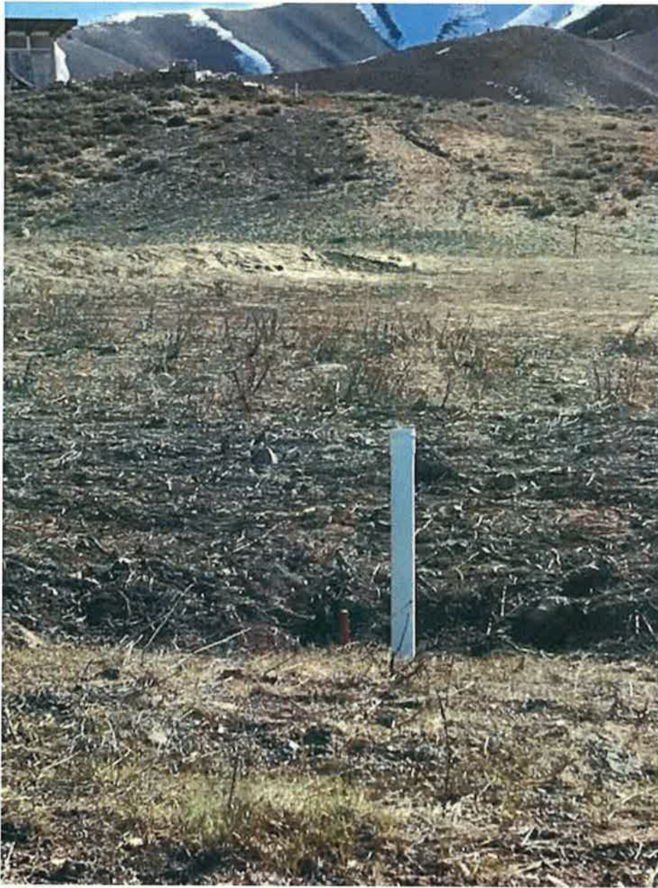
Example of stubbed in service line
