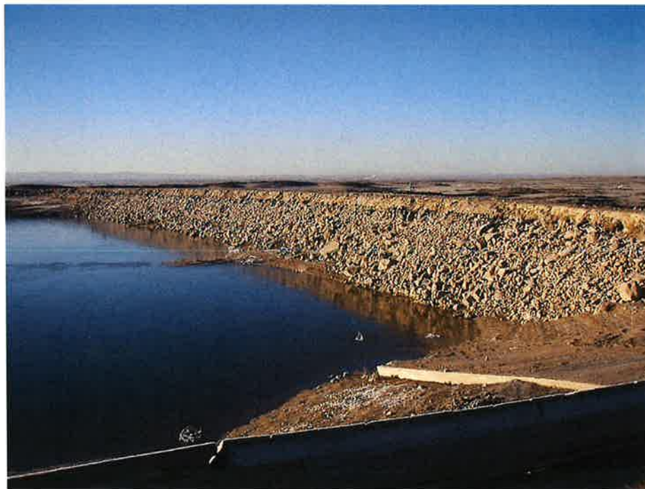
Figure 2: Looking south across west dam
