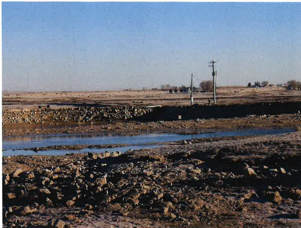
Figure 3: North POD, pump station left of power pole
