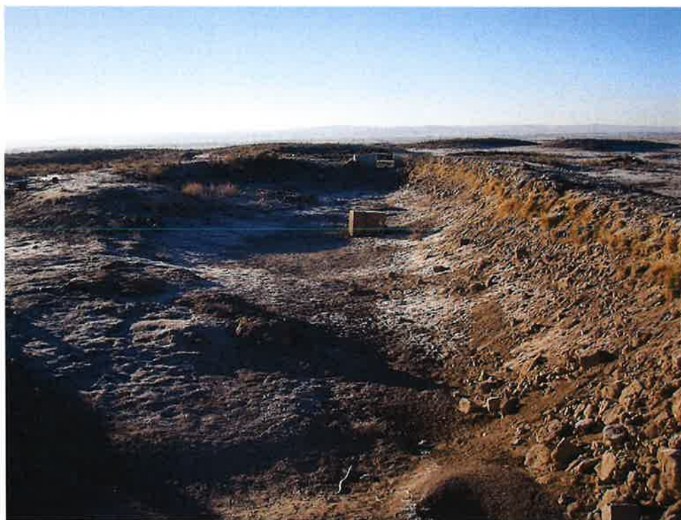
Figure 4: Looking south across spillway bay on southwest side of reservoir.
