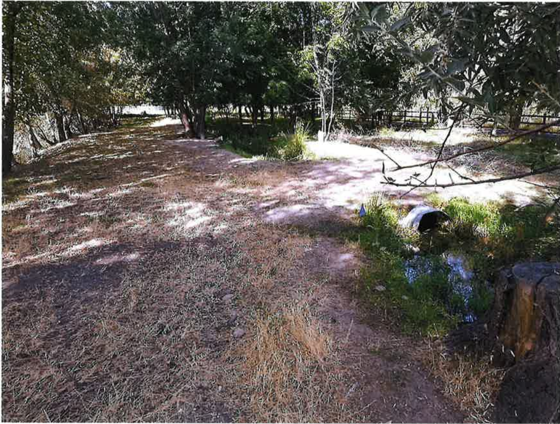
Looking West along Canal Access Road and at Crossing Culvert. Also Location of Mitigation Pipe.
