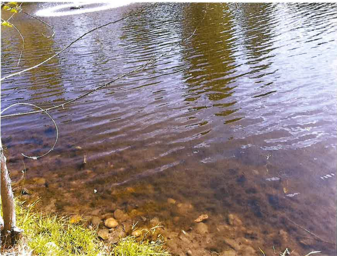
Looking at 1:1 Side Slopes of Pond (Same Slope for Entire Pond)
