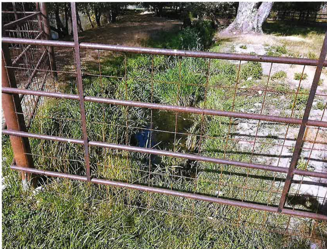
Looking West from Front Entrance at Mace-Catlin Ditch
