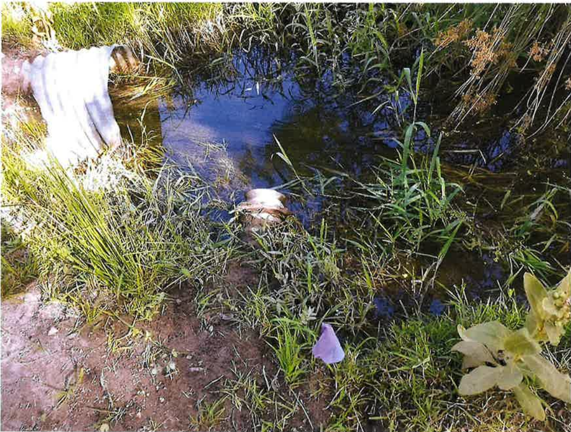
Looking at Canal Crossing Culvert (Large CMP Pipe) and Mitigation Pipe (Small CMP Pipe)
