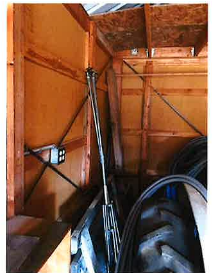
Two rain bird sprinklers used to irrigate.
