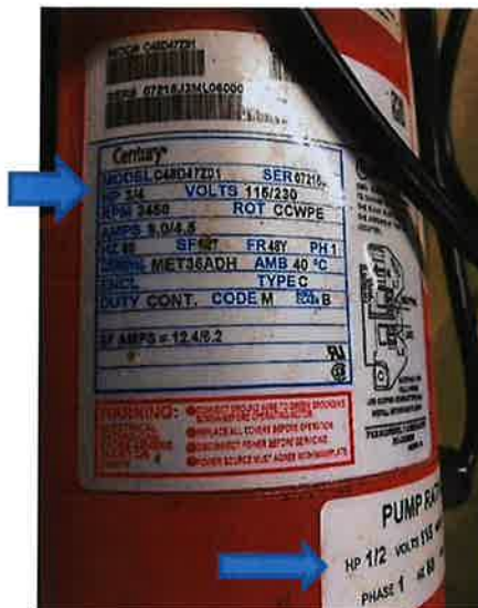
This is a 1/2 hp pump, even though the labels do not match.
