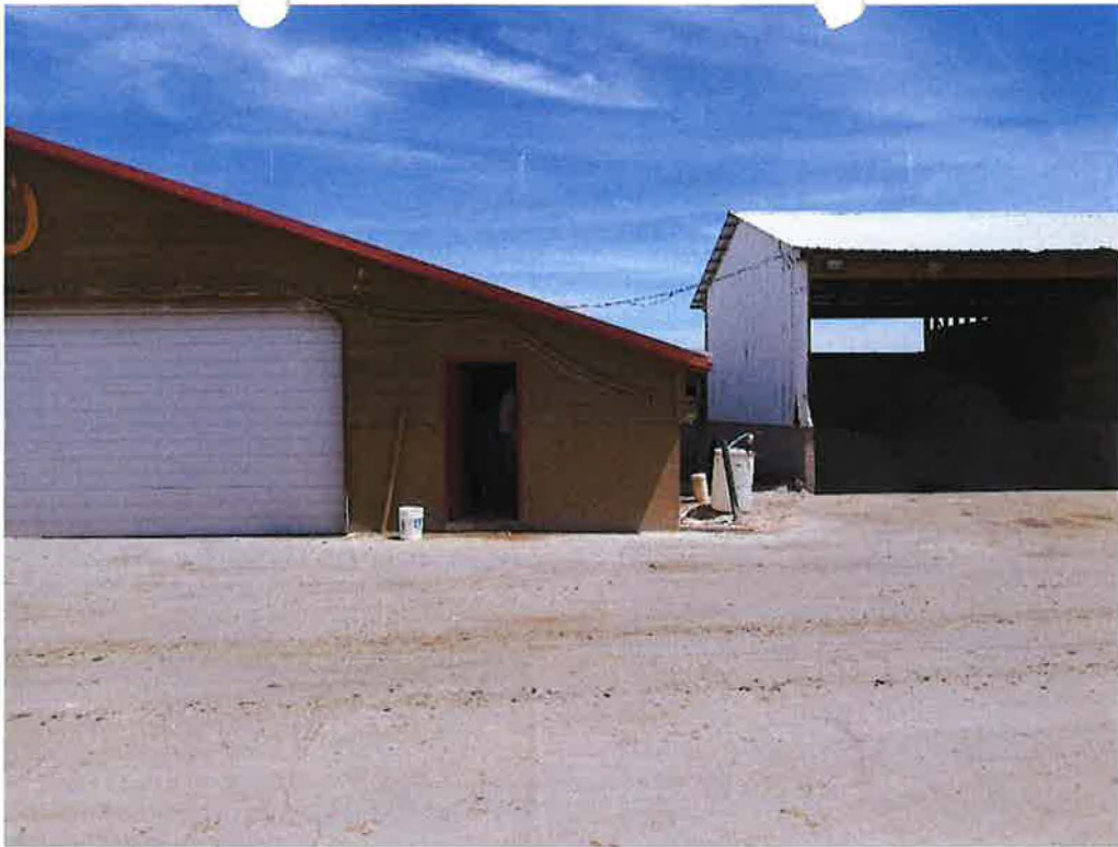
Picture 3 Well #1 Located in the Building and Well #2 Located between Building and Storage Shed
