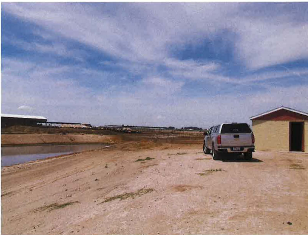
Picture 4 Building Housing Well #3
