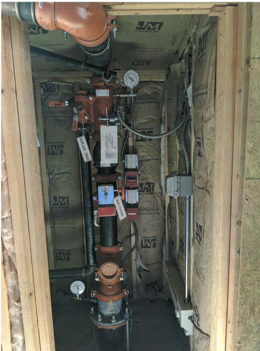
Typical Building Fire Protection Control
