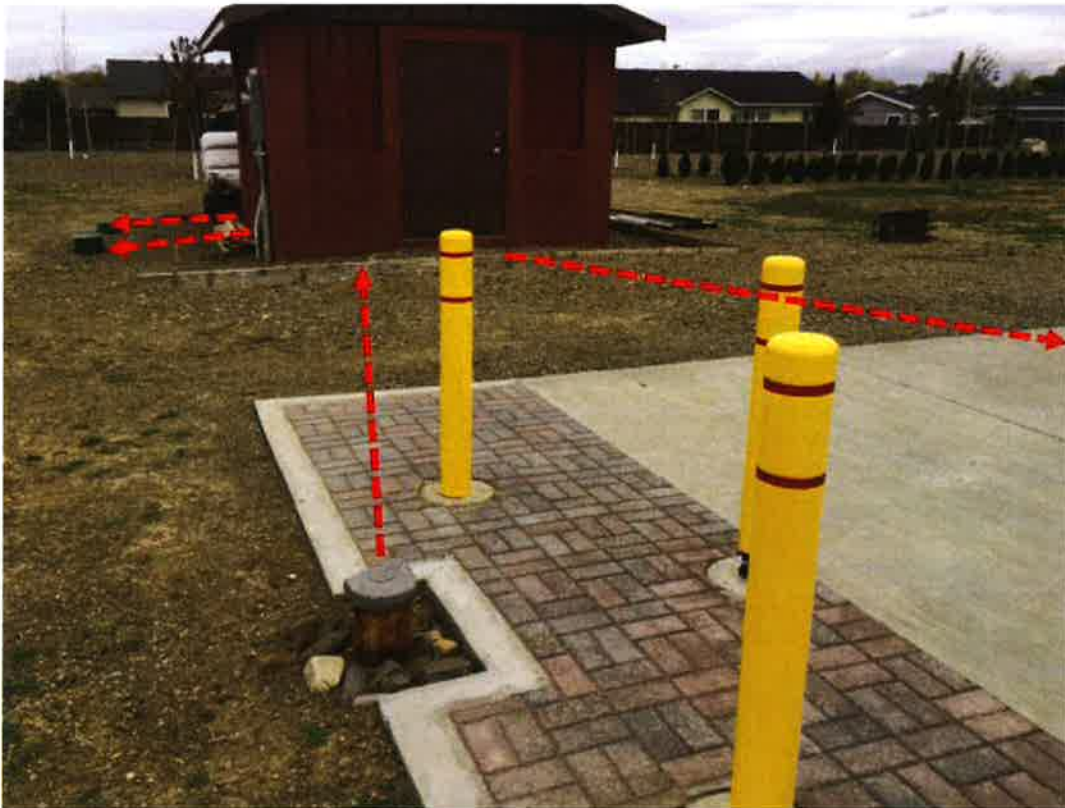
Well, with pump house in background. Dotted line shows approximate location of buried water line from well to pump house, and buried water lines from pump house to car wash and drip irrigation.
