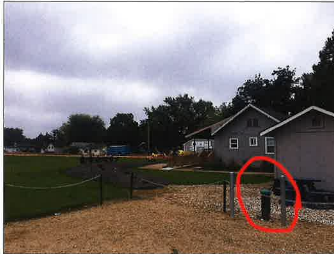
Figure 1: Point of diversion circled. Pump house is behind the picnic table.
