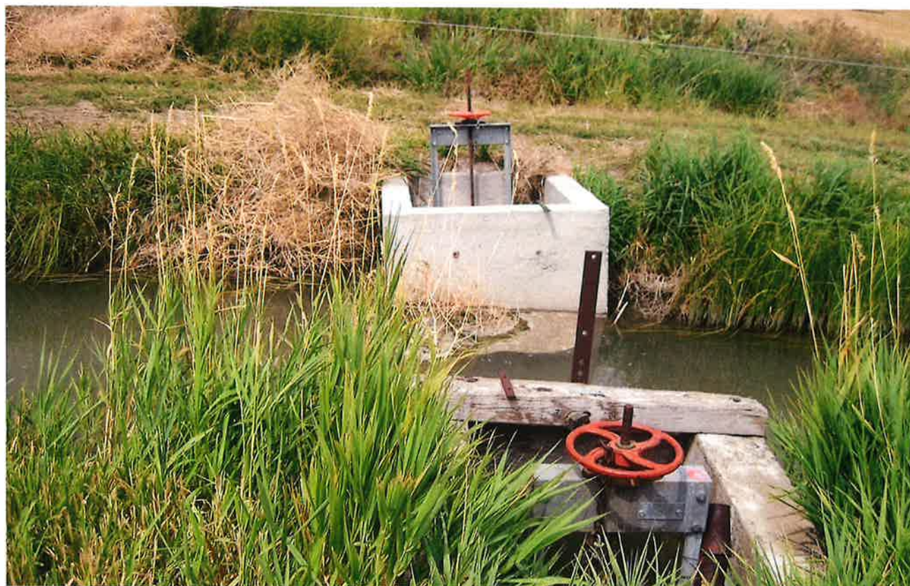
Below: Head gate into Pond
