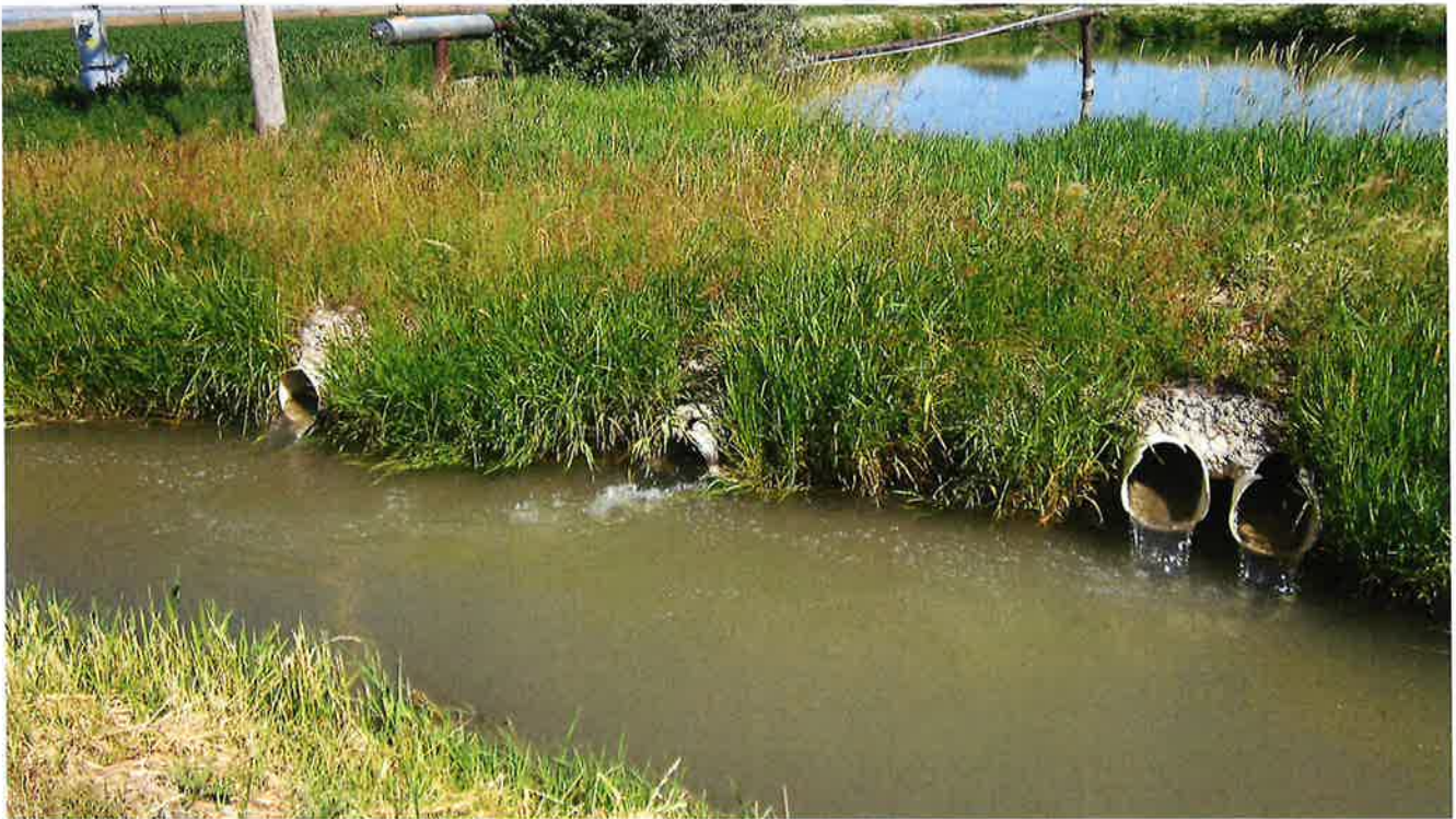
Return Flow from Pond to Lateral
