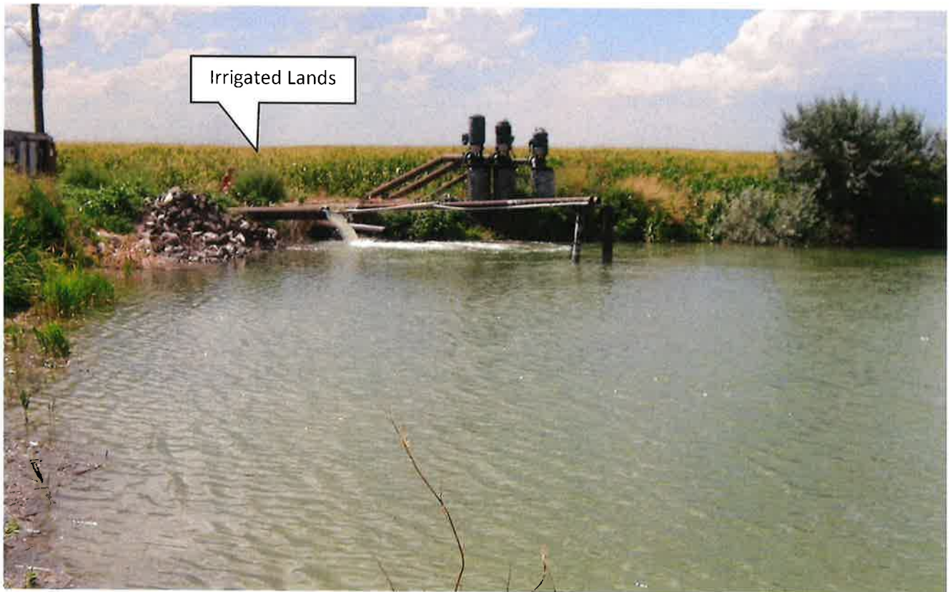
Below: Diversion to Secondary Pond & re-lift pumps
