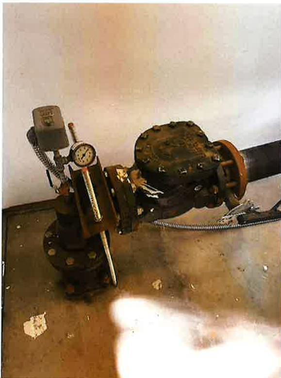
The well water exits the well house through the concrete floor on the west side of the building.
