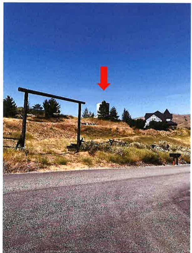
Storage tank near entrance off Highway 55.
