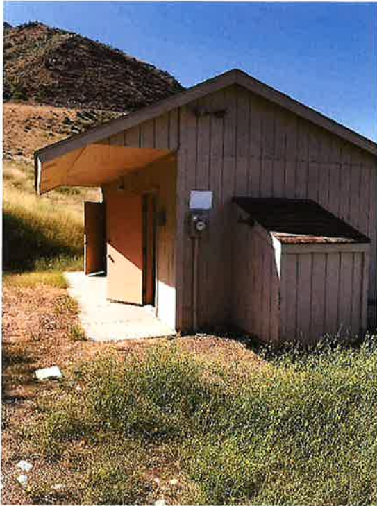
Well house looking south.
