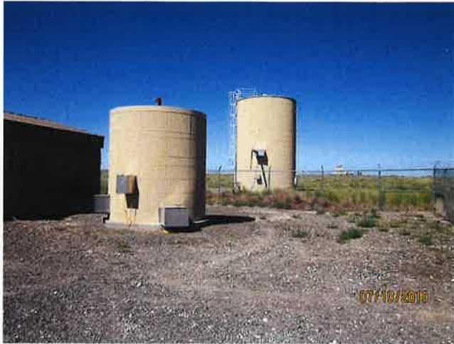
Figure 7. Tanks at the Juniper Butte Range Station that are filled with water transported from the well. The smaller tank in front is the 6,000 gal. tank used for domestic and industrial associated with this right.
