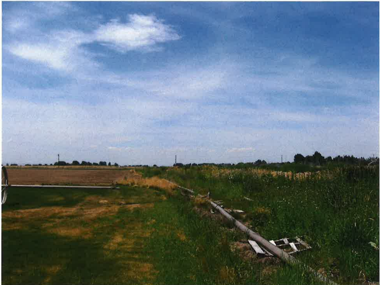
The mainline after a 90 degree turn heading toward Eagle Road along the north end of the 30 acres irrigated water permit 63-34284.
