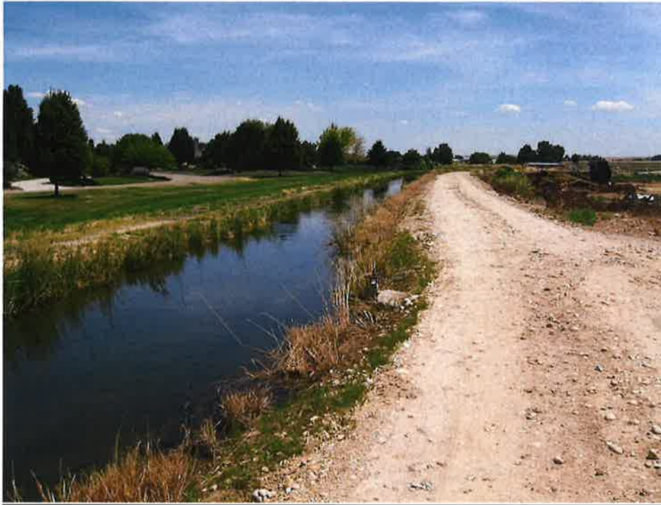
(Above) The Farr lateral with the farm headgate shown in the center right of the picture.
