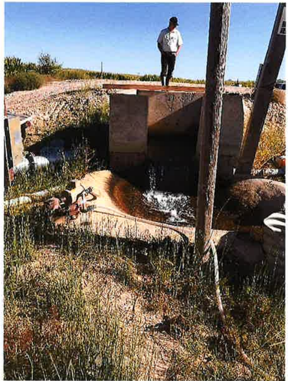
Regulation pond is behind the concrete structure. Pump to the large pivot is on the left. Small red pump on left supplies water to the non-pivot areas.
