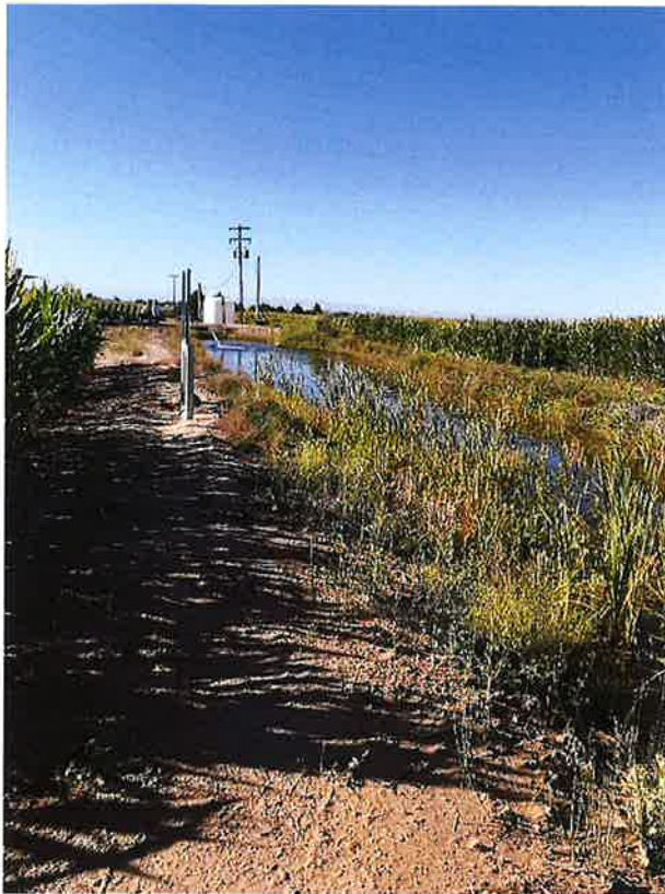
Irrigation regulation pond.
