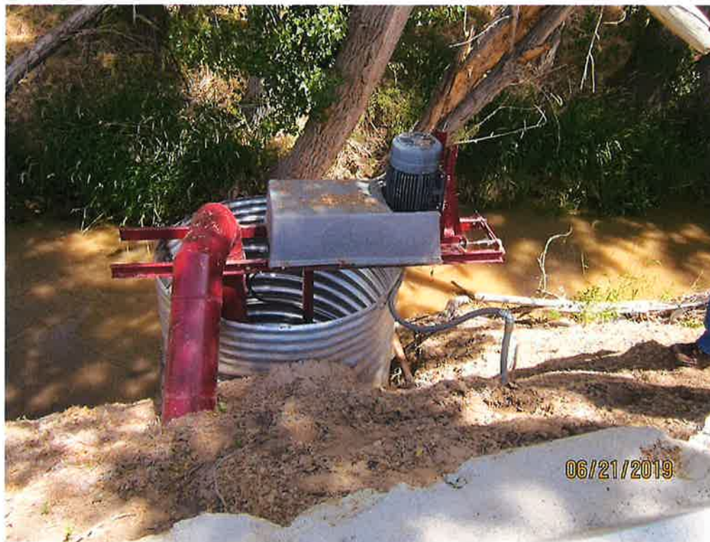
Parma low-lift pump (POD) capable of diverting 3.08 cfs out of Conway Gulch (above) into the stilling basin (below). Surface water from Farmers Cooperative Irrigation Ditch Company is also diverted using gravity flow into the stilling pond, through submerged outlet pipes.
