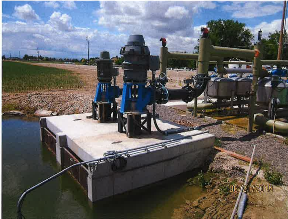
Two AMP re-lift pumps (above) diverting water from the stilling basin to pressurize the irrigation system. Excess irrigation water returns to Conway Gulch drain via the weir shown below.
