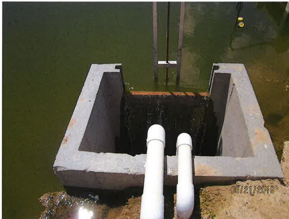
Two AMP re-lift pumps (above) diverting water from the stilling basin to pressurize the irrigation system. Excess irrigation water returns to Conway Gulch drain via the weir shown below.
