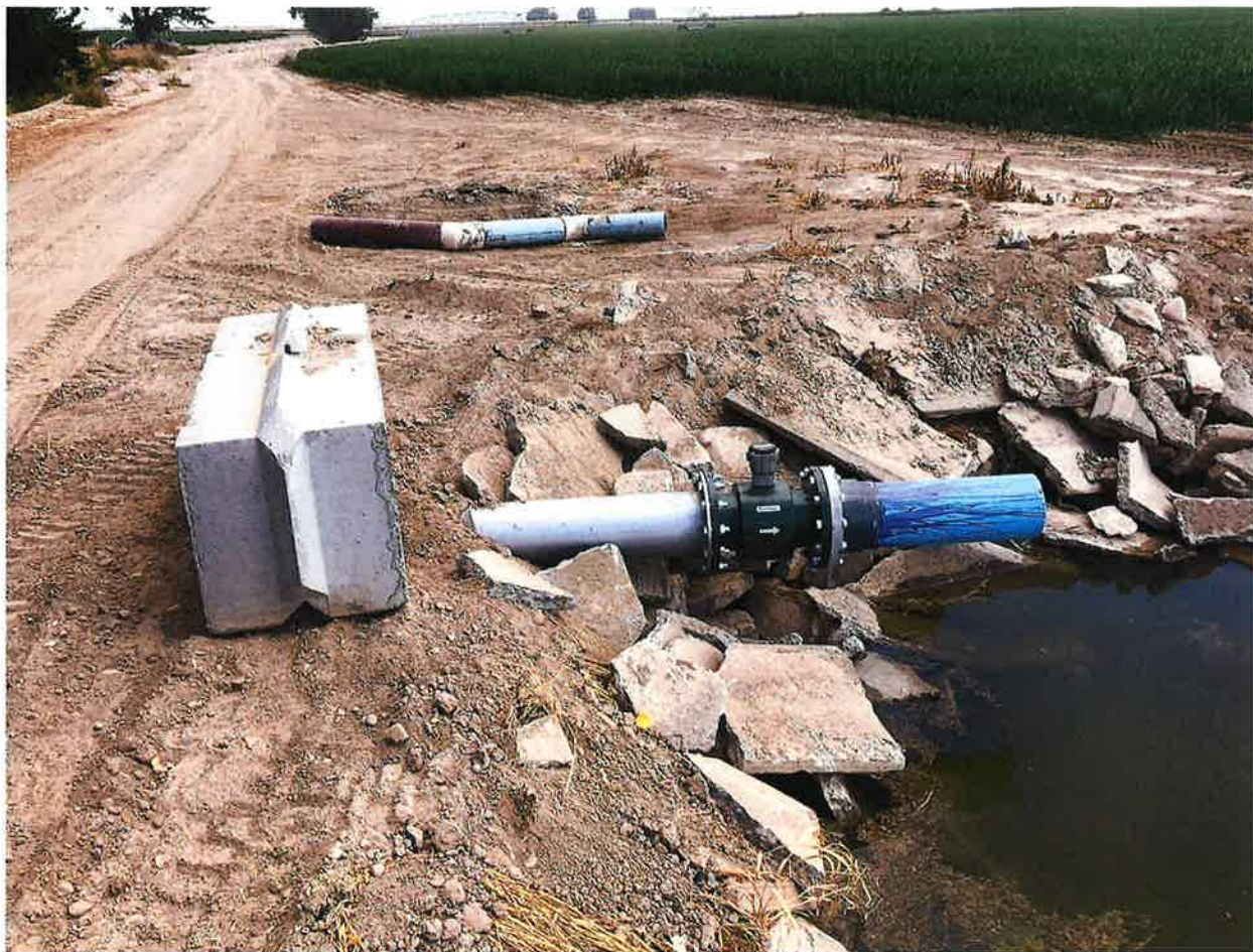
On July 29, 2019 this photo was sent to IDWR by the Watson Company to provide proof that a flow meter was installed.
