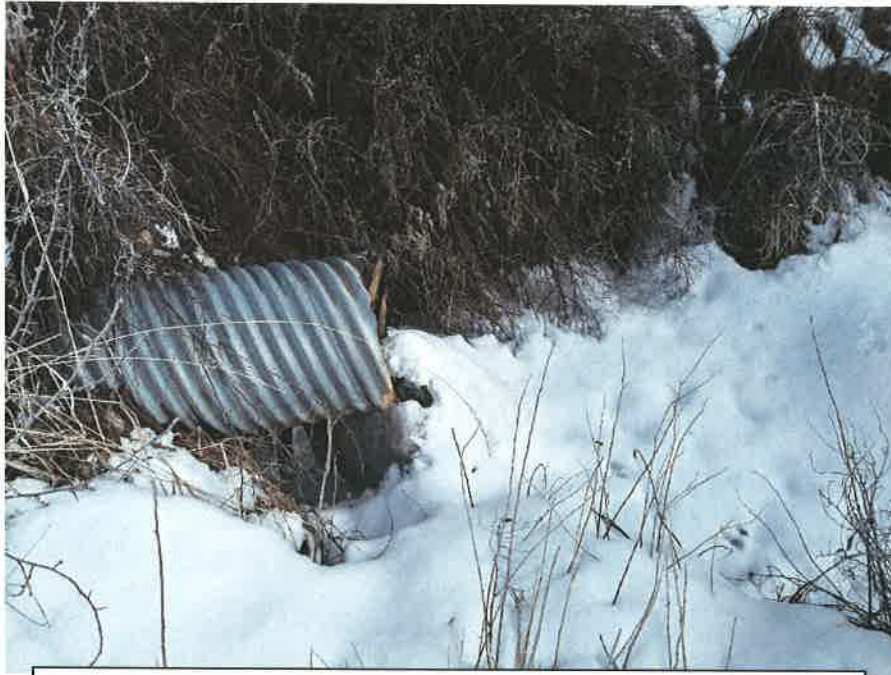
Figure 5 A culvert diverts the unnamed stream under the irrigation canal to the permit holders property. At the time of the first visit the stream was running at 40 – 60 gpm. Stream water is conveyed through the constructed ditch along with groundwater to the pond.
