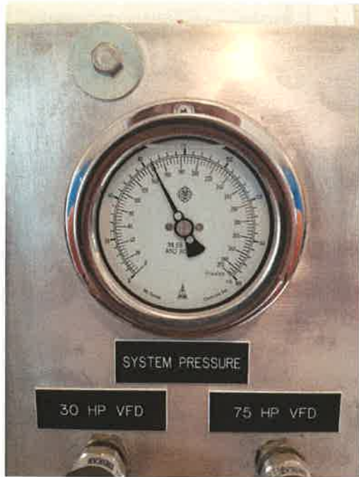
Figure 3 The system pressure gauge for the two pumps which supply water for the domestic and irrigation uses. It is my understanding from the field exam for right 63-31745 that system pressure drops to 20 psi when water is diverted from the hydrants for fighting fire.
