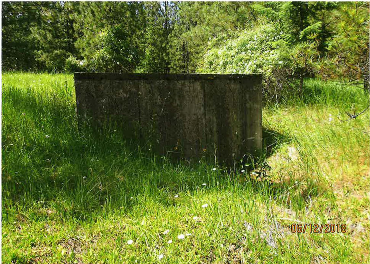
Storage tank where 5 gallon bucket test was performed and filled in 20.6 seconds.
