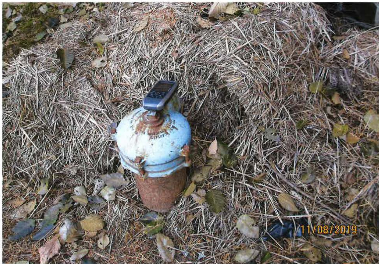
Point of diversion.
