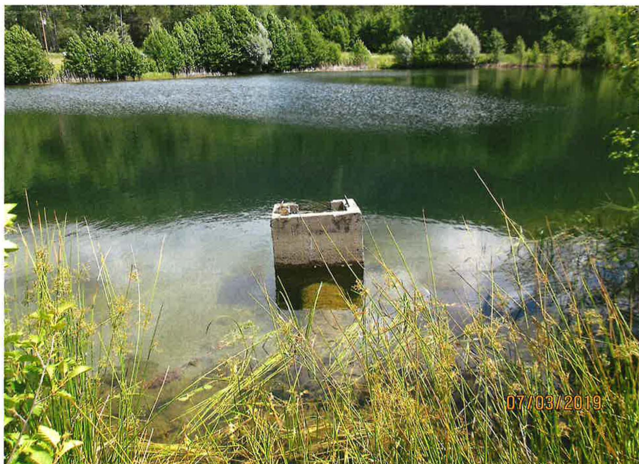
Screened outflow structure.
