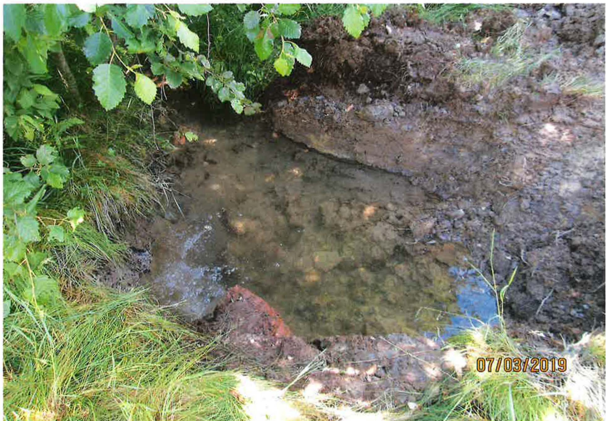
Flow from pipe into pond.
