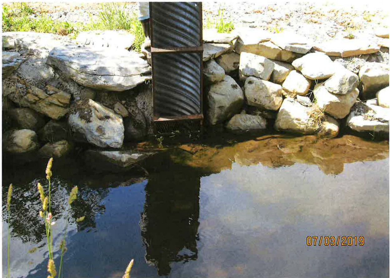
Screened diversion structure to pond.
