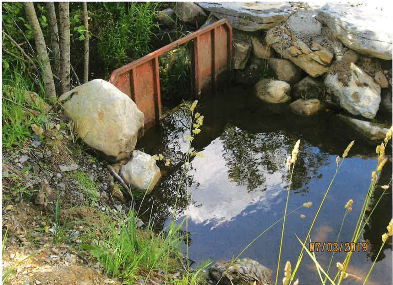
Check structure in creek for diversion pipe.
