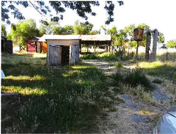
Well and pump house
