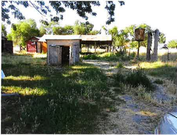
Well and pump house
