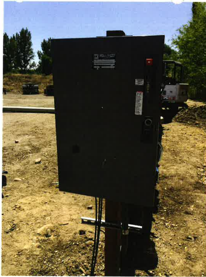
Well 2 Pump Panel. Pump is constant speed.
