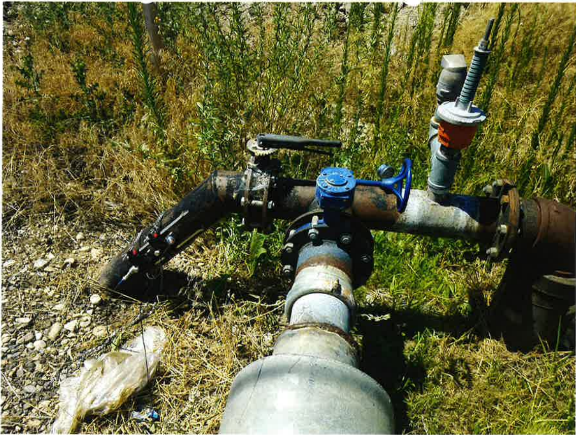
Well 1 discharge piping with portable flow meter attached
