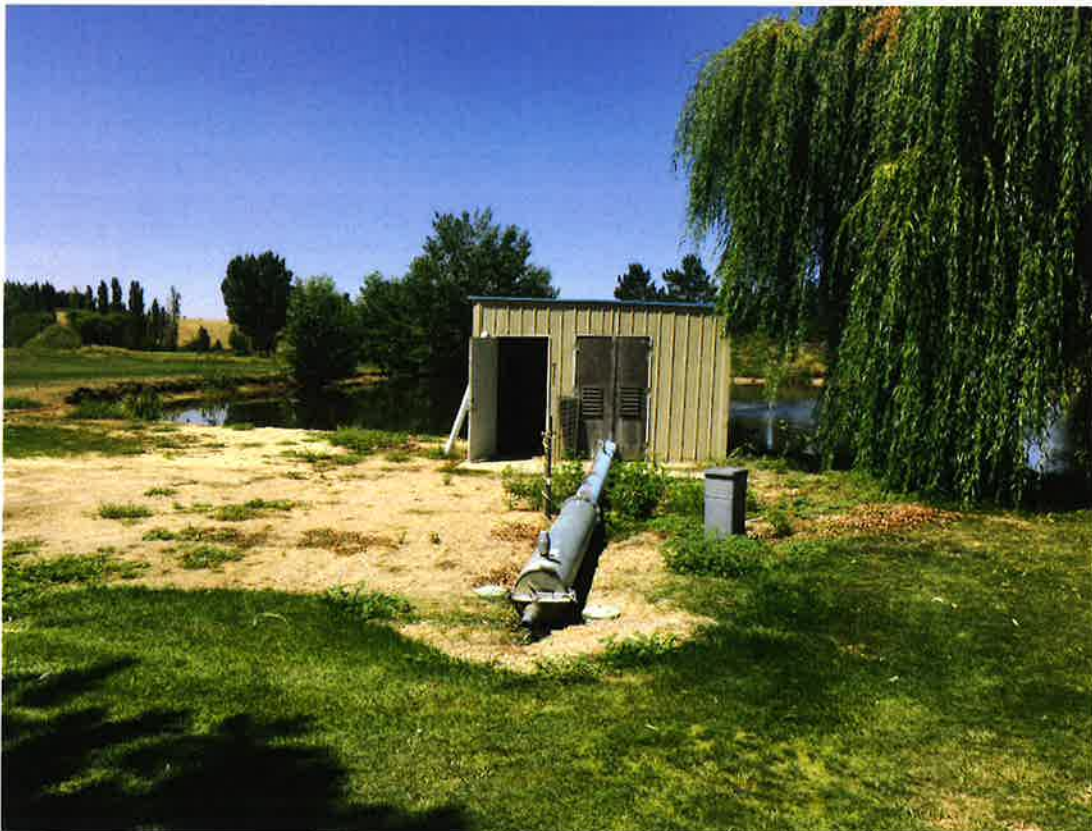
Pressure irrigation pump station with discharge pipe and filter (foreground) looking west. Water from Well 2 enters the pond through an open channel at far side of the pond.
