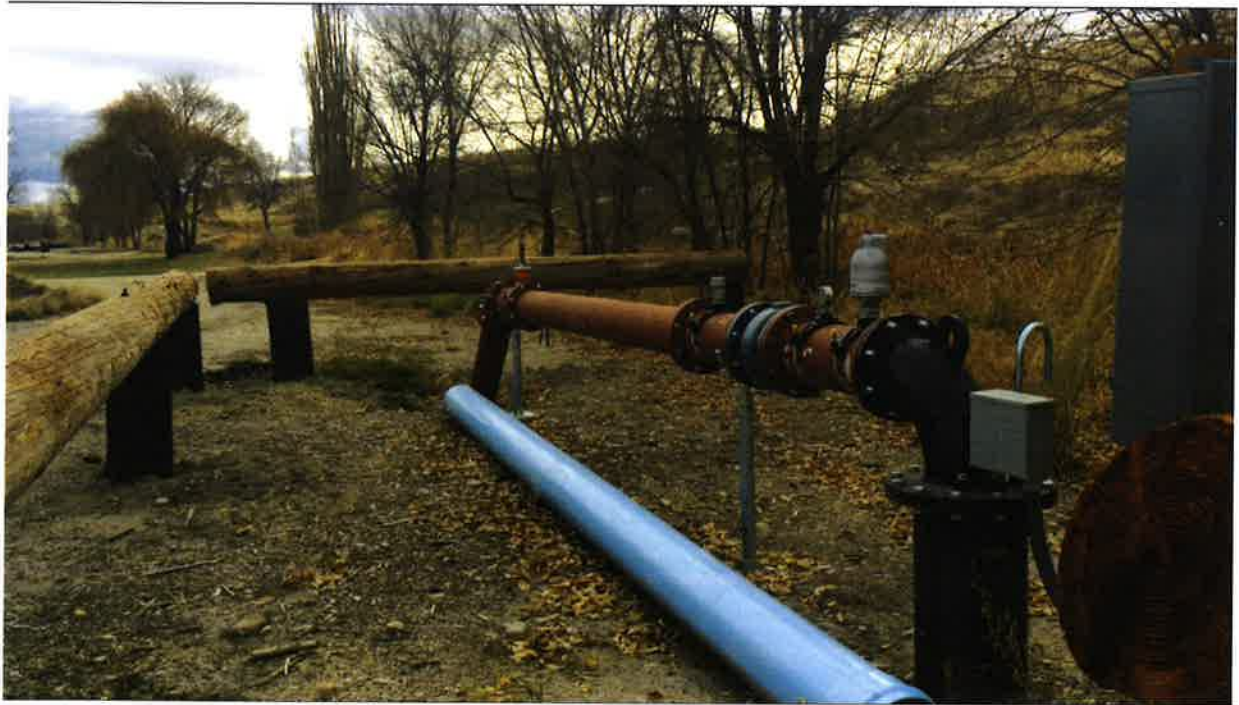
Well 2 and discharge piping. Mechanical piping appurtenances (from right to left) include discharge elbow, air/vacuum valve, pressure gage, check valve, 2-inch ball valve for winterization, straight spool for future flow meter, pressure relief valve, and butterfly valve (not visible, but located immediately past pressure relief valve).
