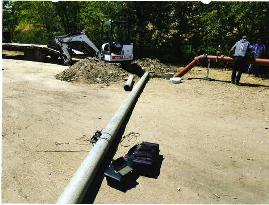
Temporary 10-inch aluminum mainline (as of 7/23/2018), prior to installation of permanent buried mainline. Portable ultrasonic flow meter used for flow measurement shown on pipe.
