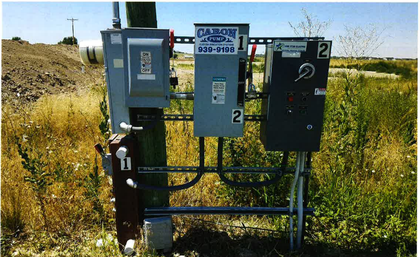
Well 1 pump controls. Controls for unrelated surface water pump also.
