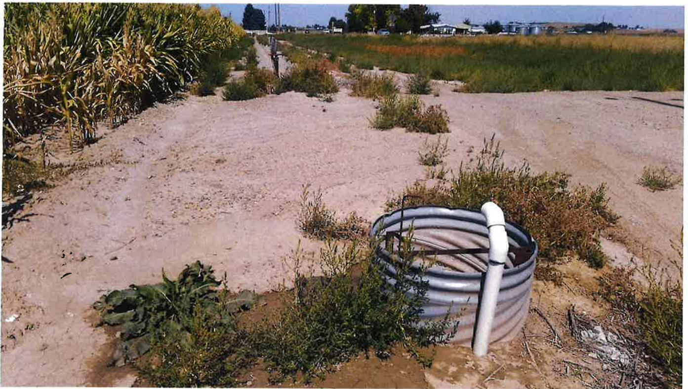
Ditch and head gates in supplying SE corner of place of use.
