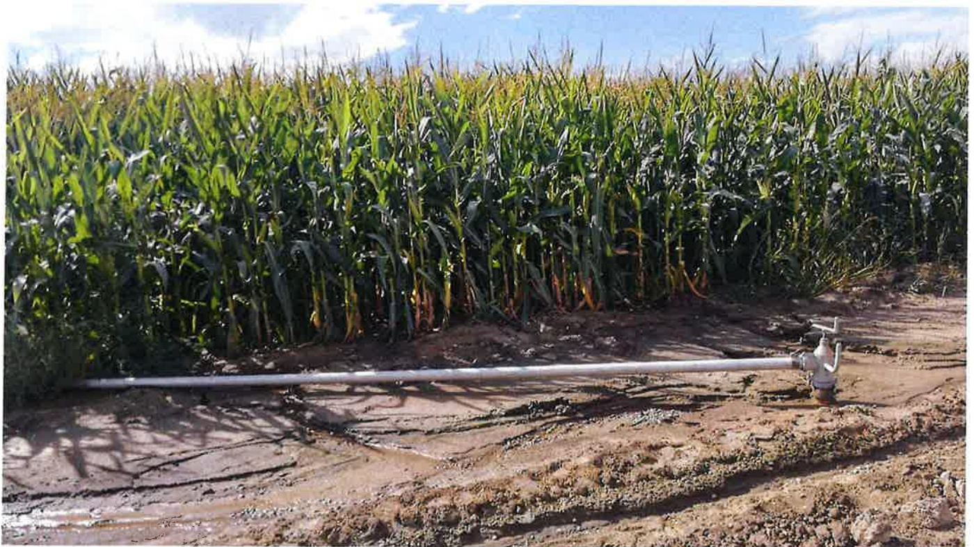
One riser to the NE corner from POD 935523.
