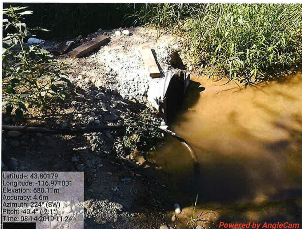
POD 935524: Unnamed drain water enters a stilling structure. Flow is to the left.
