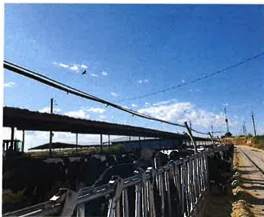
Water line for Misters along top edge cow pen
