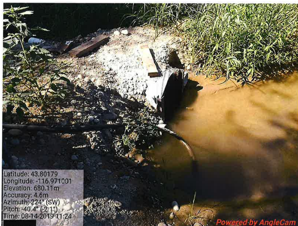
POD 935524: Unnamed drain water enters a stilling structure. Flow is to the left.
