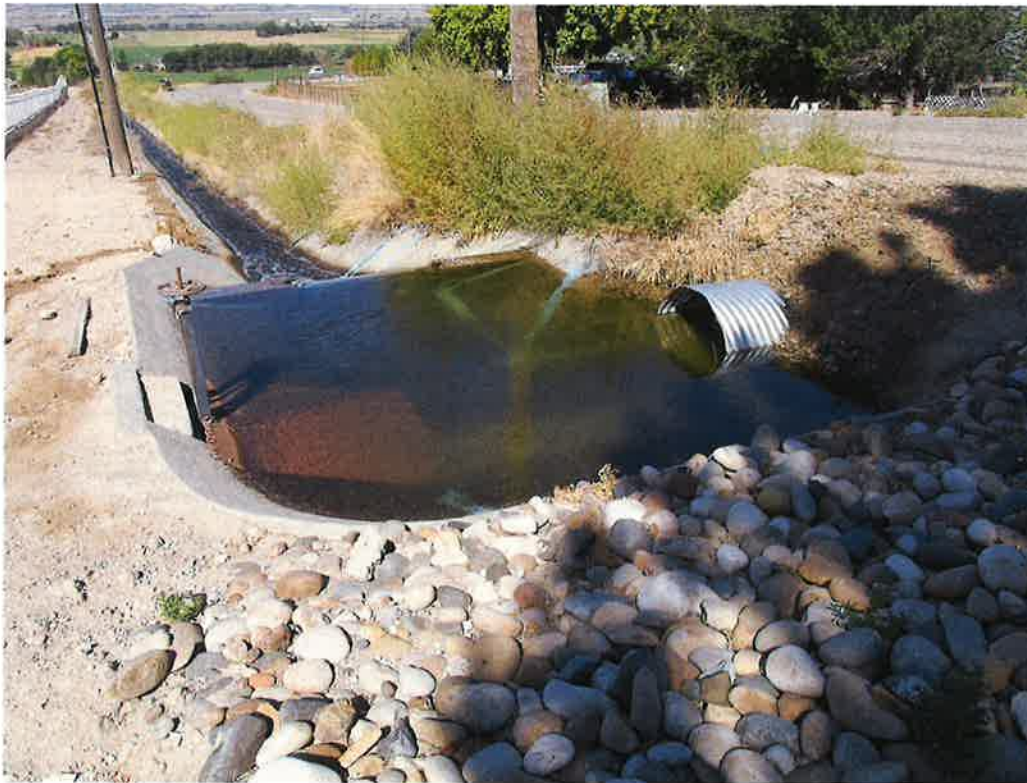
Surface water delivered from Black Canyon Irrigation District. The headgate to the subdivision is at the left side of the pool almost directly across from the culvert.
