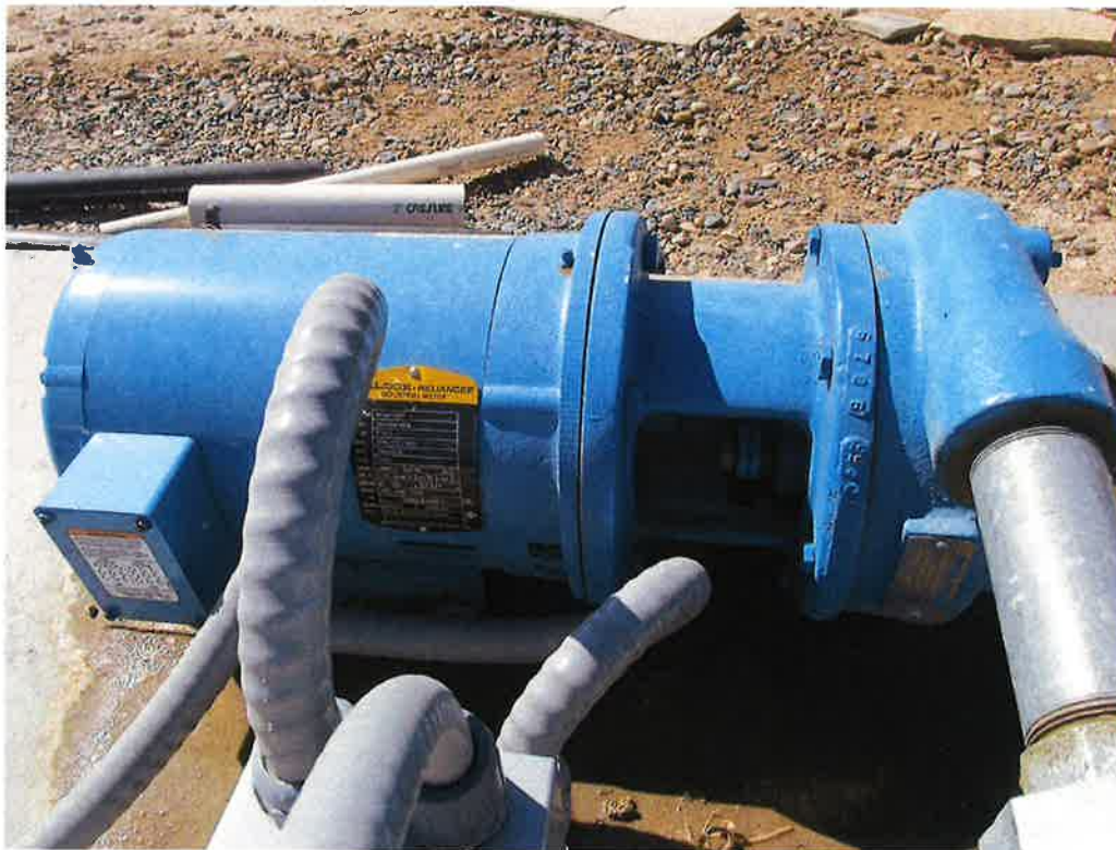
7.5 hp pump used to pressurize the surface water irrigation system.
