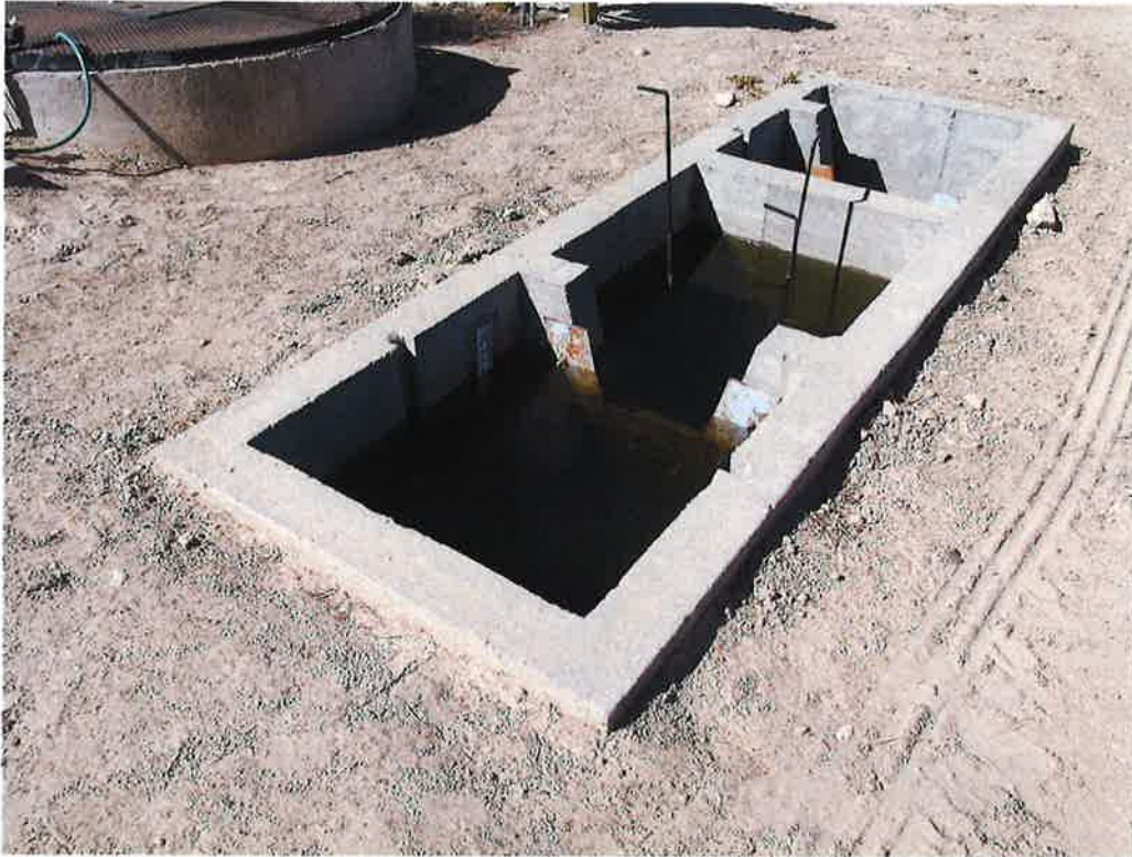
Surface water control box with two headgates. The closest headgate (with staff gage) sends water to the circular tank in the left corner from which the surface water is pumped and delivered to the subdivision via a 7.5 hp pump. The far headgate (which also has a staff gage) delivers water to a downstream (or down gradient) neighbor.
