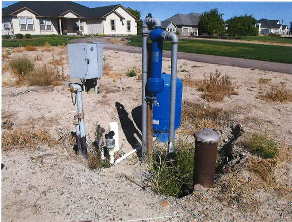
Groundwater well and electrical control box for Eagle View Estates.
