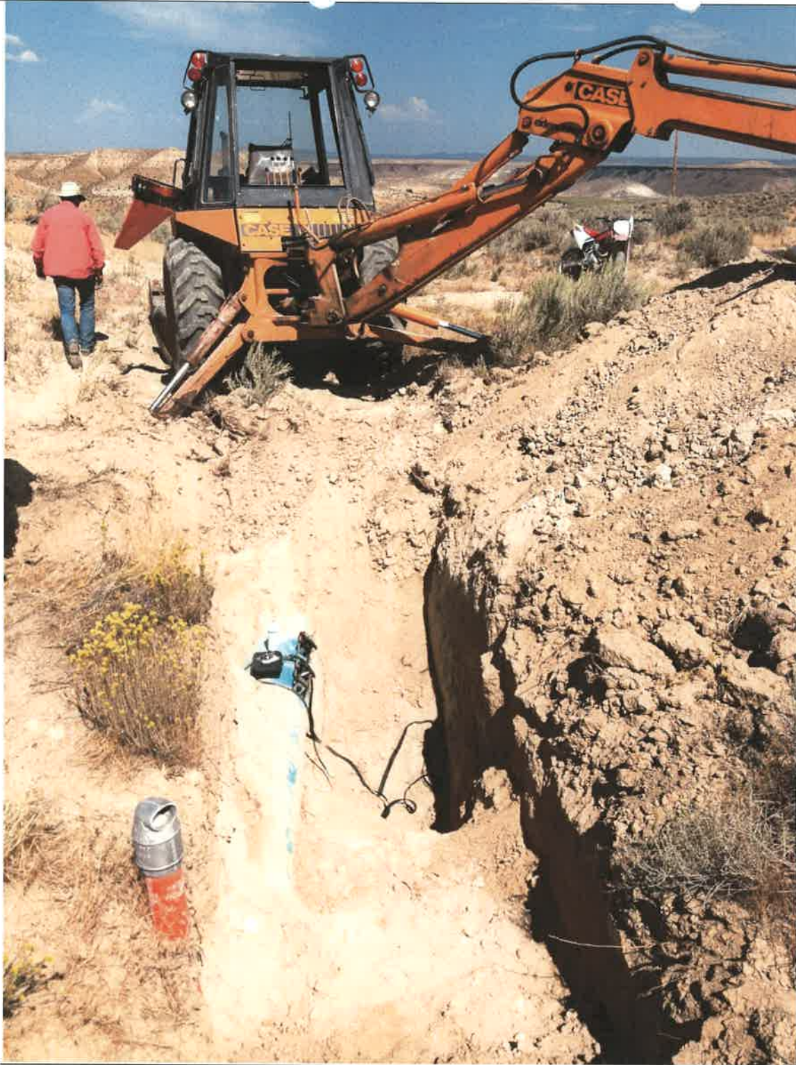
Excavated portion of pipe ~100 feet of lift above well. (topo map)
