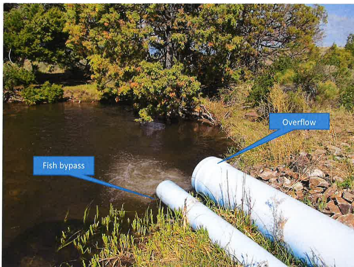
Photo 3: Fish bypass and overflow returning to Hawley Creek
