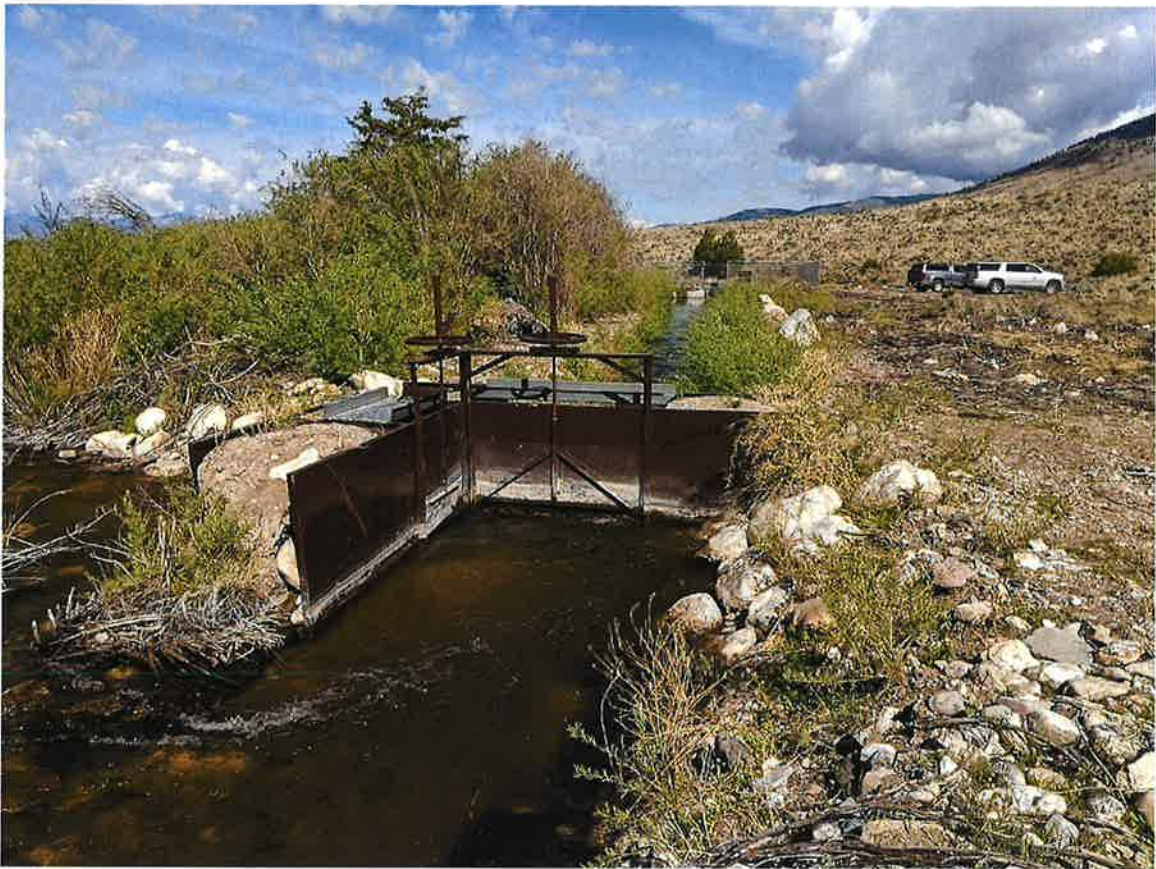
Photo 1: Diversion on Hawley Creek
