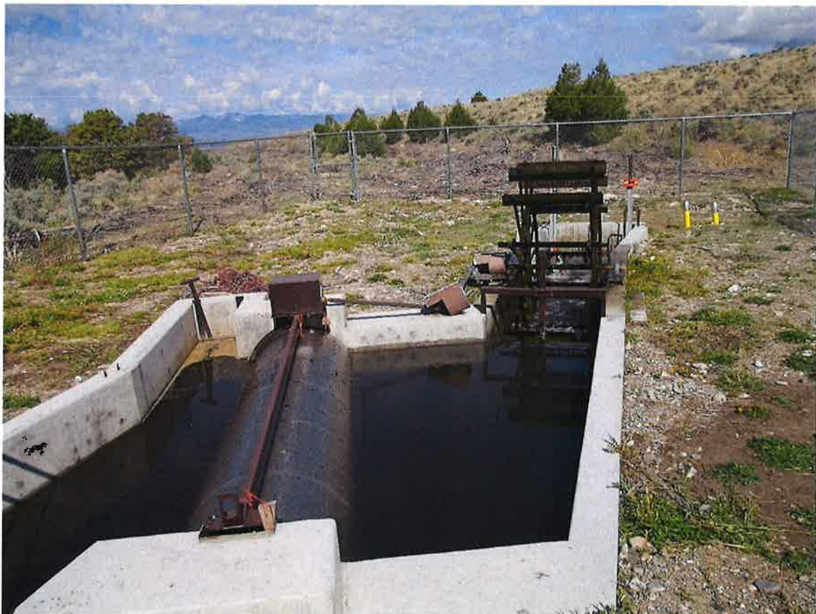
Photo 2: Overview of fish screen structure
