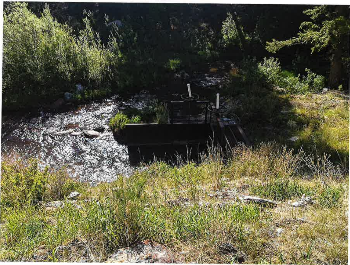
Photo 1: Diversion on Hawley Creek
