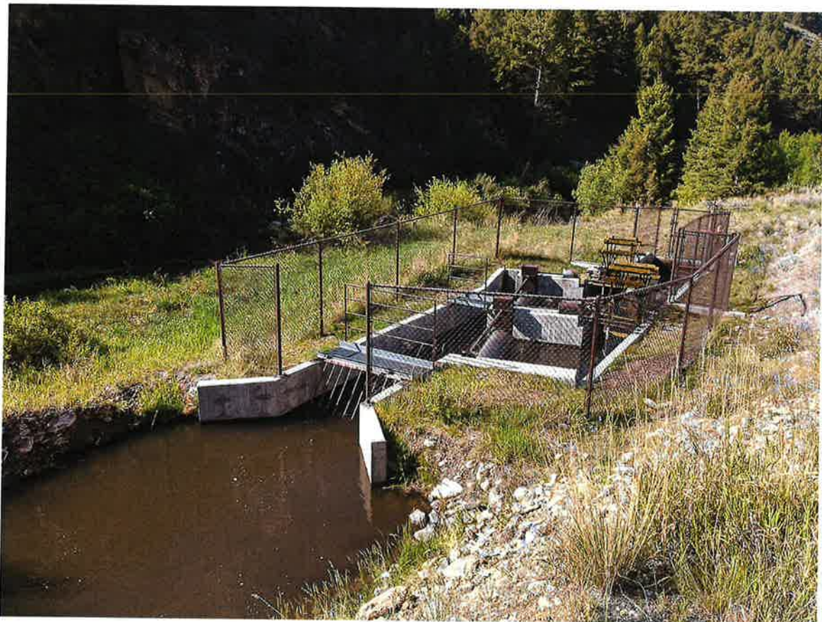
Photo 2: Overview of fish screen structure
