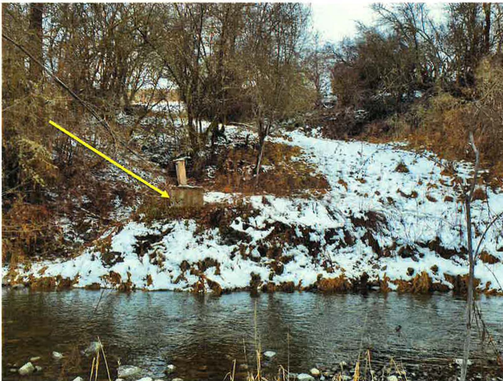
Figure 3. Picture of spring structure – circular cement structure with power supply box. Approximately 3 feet of structure is above ground, the remaining 17 feet is buried.
