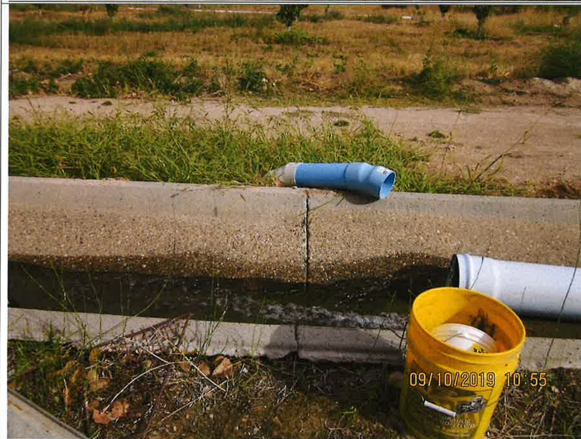
Figure 8. Secondary discharge into concrete ditch for delivery to other fields.
