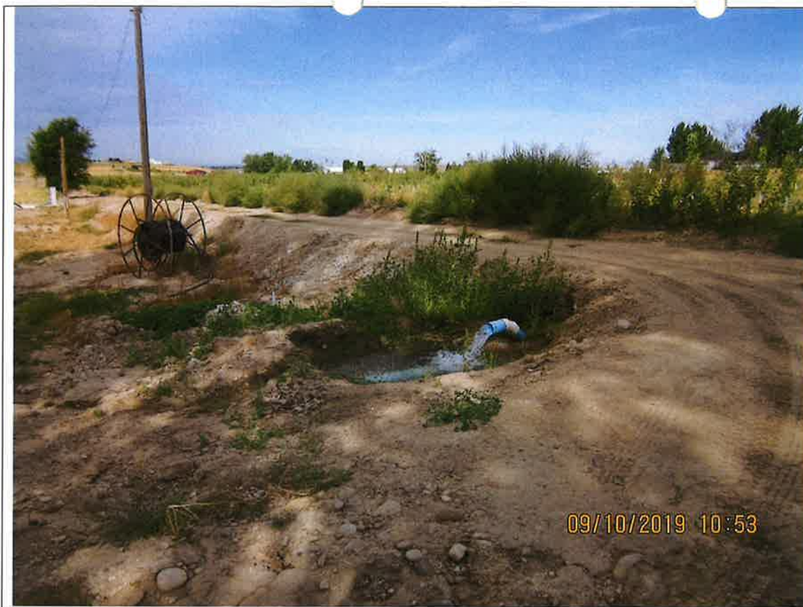
Figure 7. Well open discharging into collection basin.
