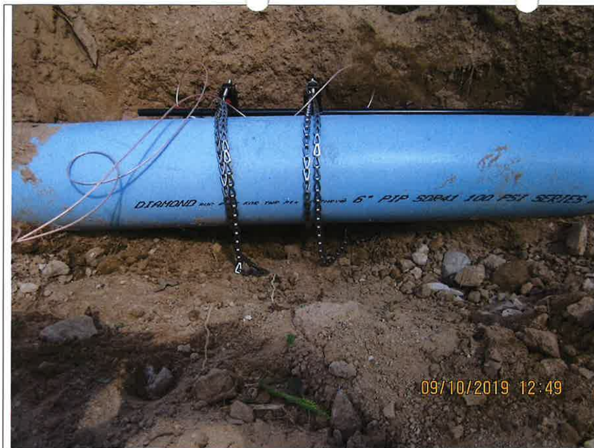
Figure 10. Measurement taken on Diamond 6 inch SDR 41100PSI PVC plastic irrigation pipe.
