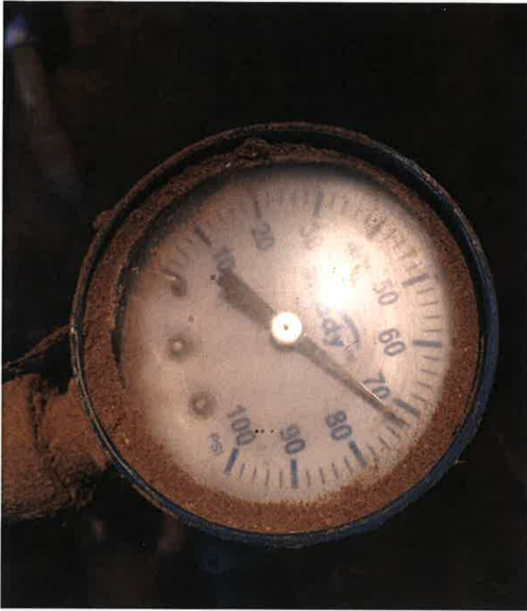
Figure 3 The system pressure for the dairy is held at 70 psi. Both wells are connected to the same system to the pressure is equal for both.
