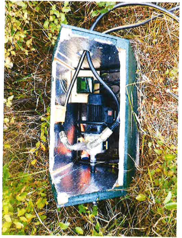
Pump House holding 1 hp Sprinkler Pump with timer drawing water from the Middlefork of the Payette. Distributes water via two hose pipes to above ground sprinklers per original application.
