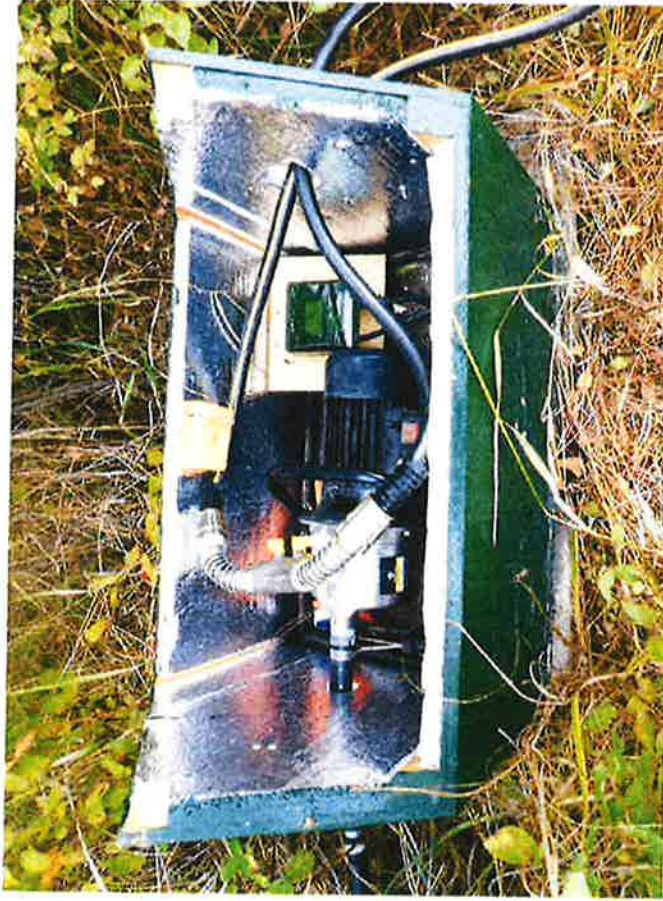
Pump House holding 1 hp Sprinkler Pump with timer drawing water from the Middlefork of the Payette. Distributes water via two hose pipes to above ground sprinklers per original application.
