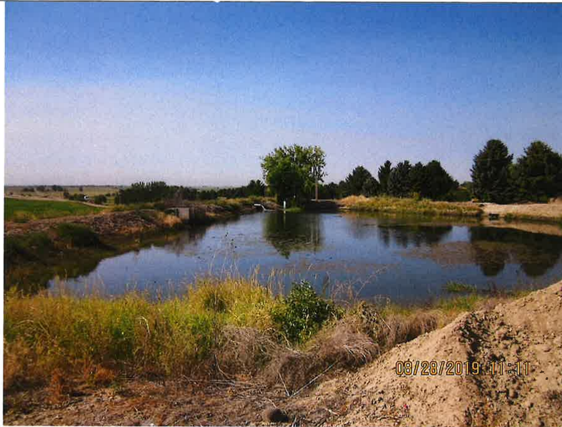
Figure 5. The 0.5 acres holding pond is approximately 8 to 10 feet deep at the deepest point.
