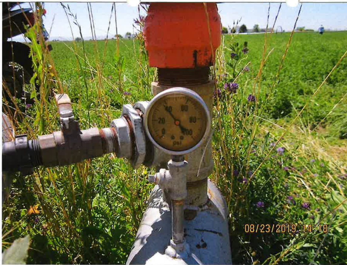
Figure 7. Pressure gage after booster pump reading about 38 psi.
