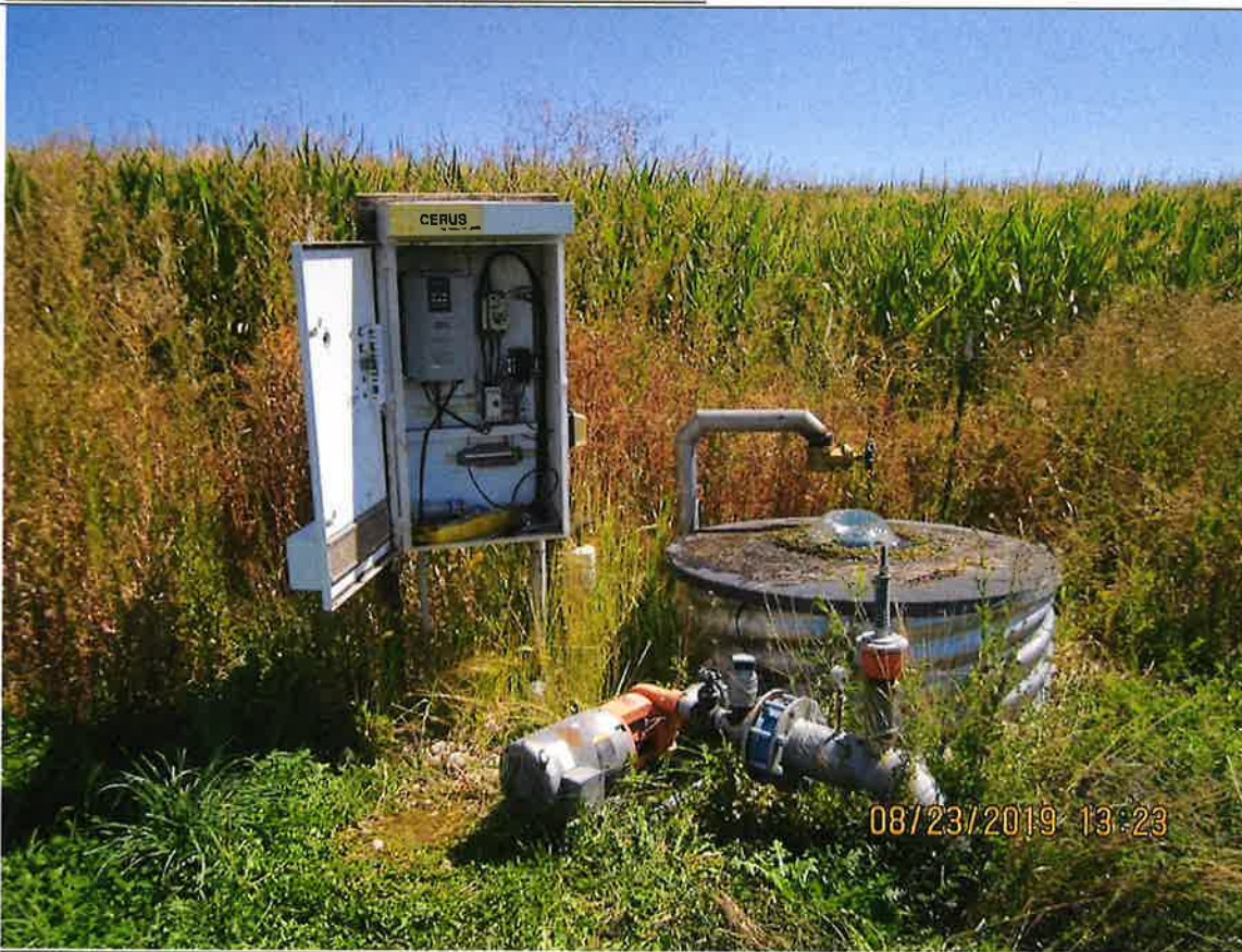
Figure 2. CMP bubbler, supply pipe from pump, control panel and booster pump from bubbler.
