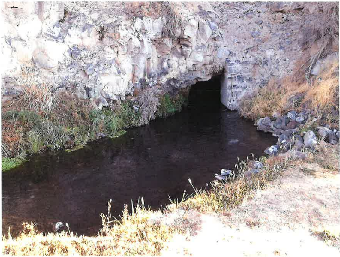
The ground water point of diversion, the constructed tunnel.
