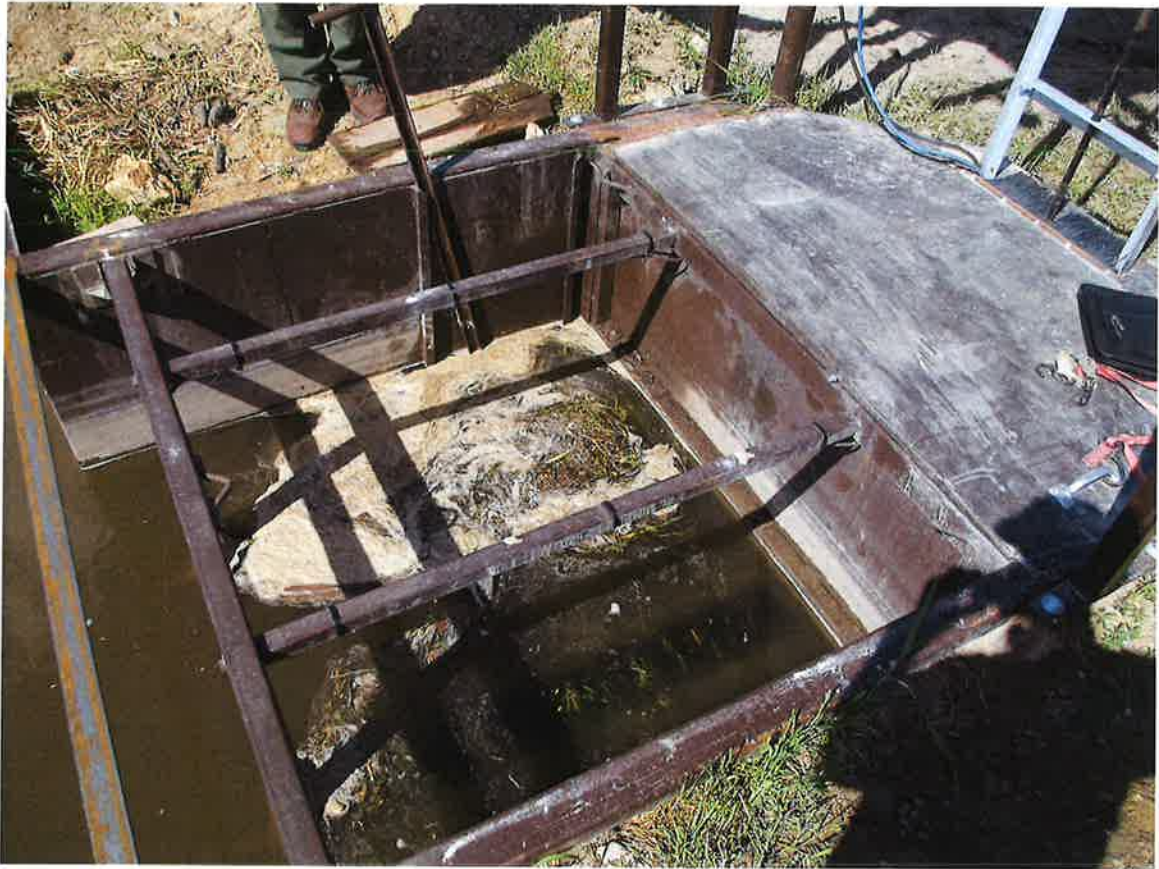
Photo 3: Close-up of fish screen structure
