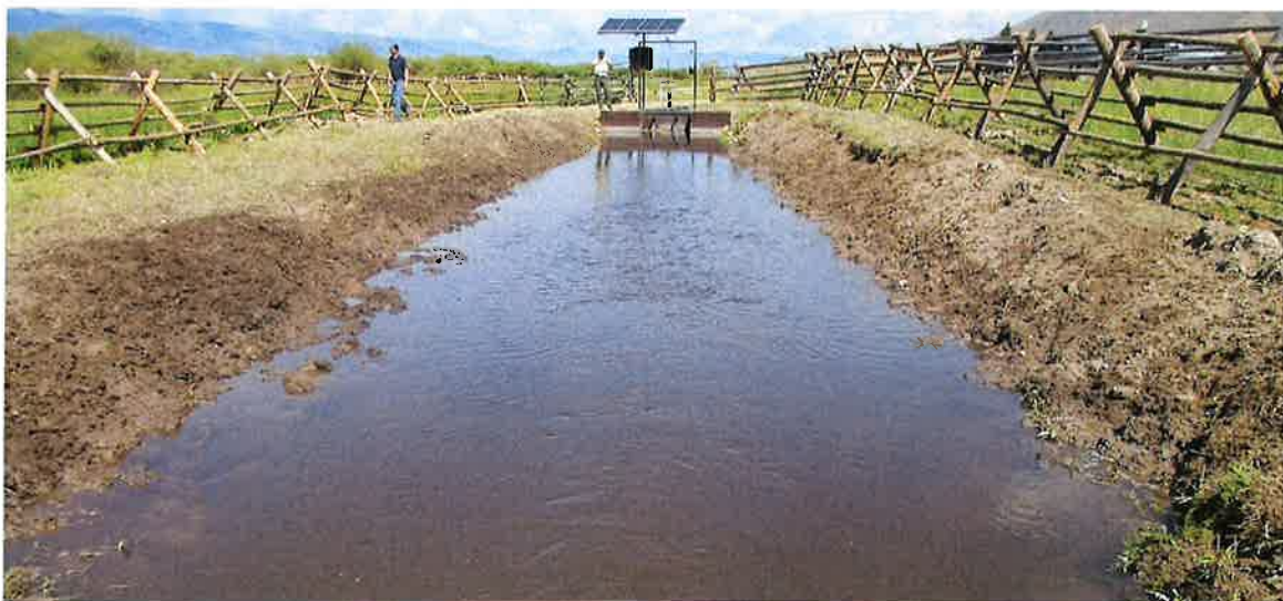
Photo 2: Fish screen/bypass approach
