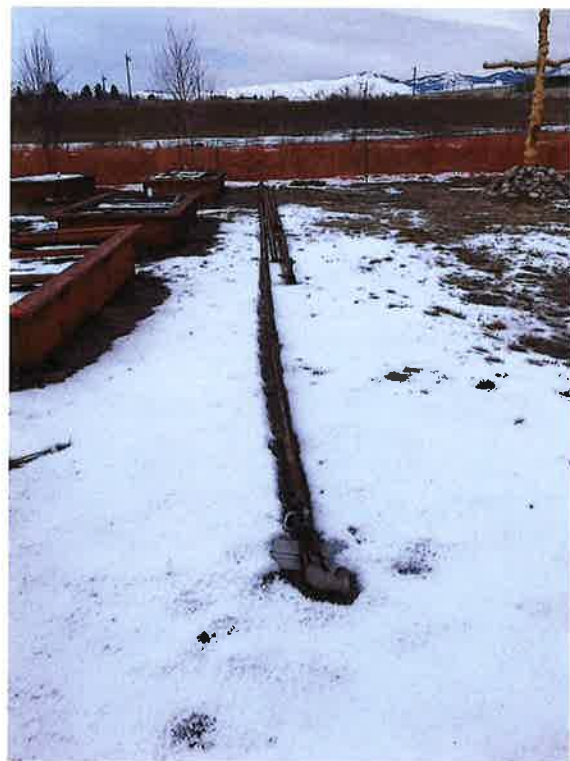
Irrigation pipe going to the vicinity of the valve. Raised beds.
