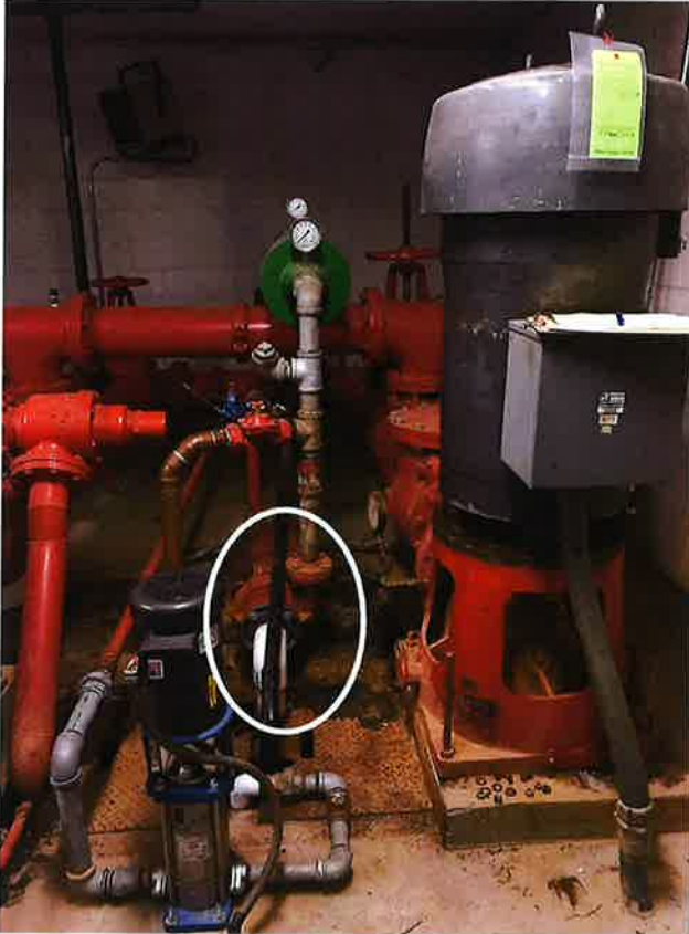
Red irrigation pump is circled above.
