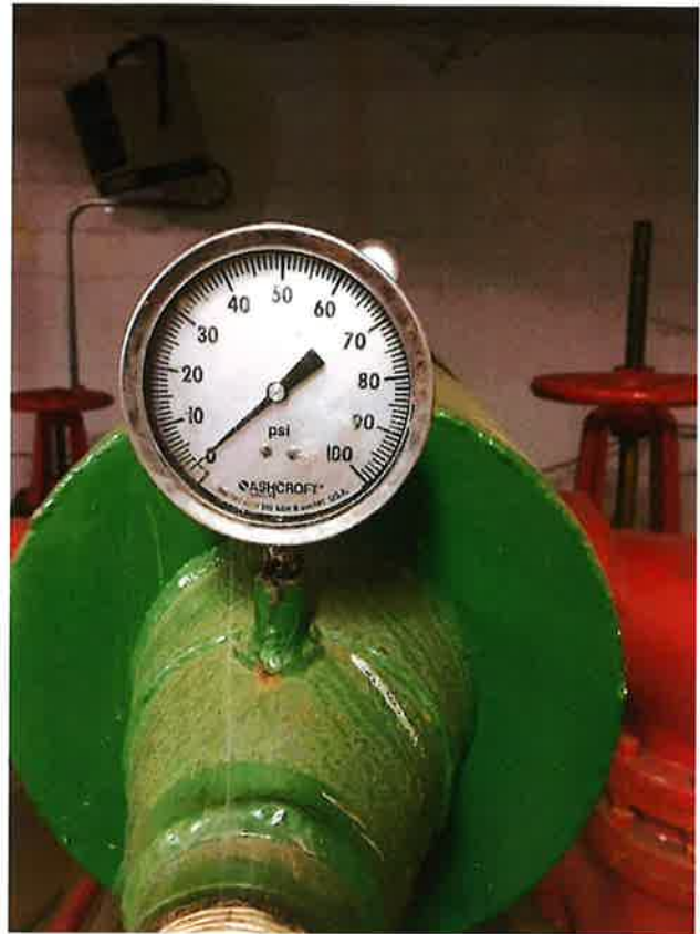
Pressure gauge on sand trap.
