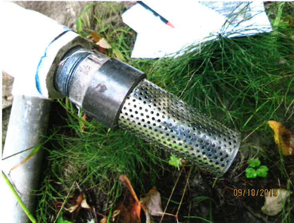
Screen intake on end of diversion pipe.
