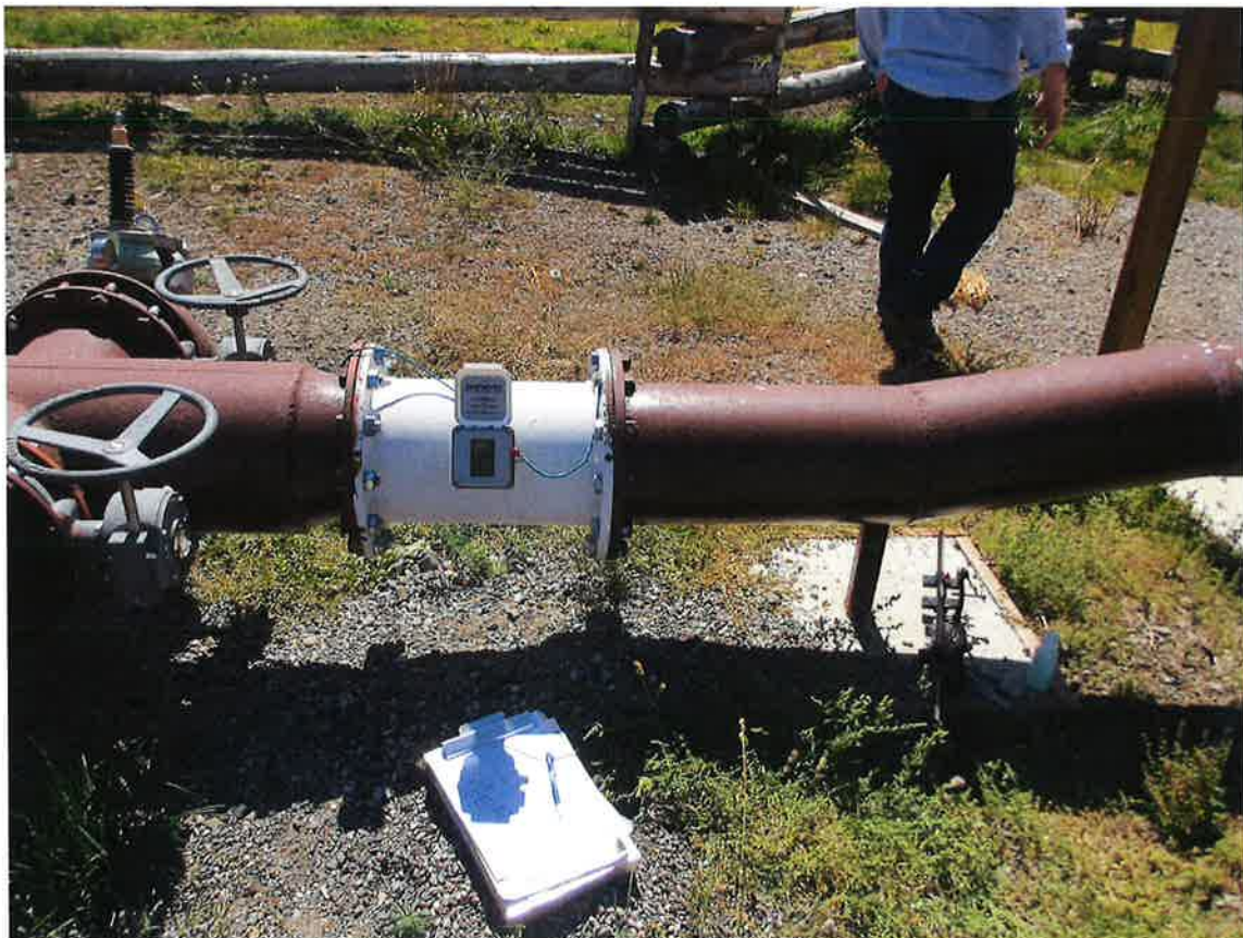
Meter installation at upper well
