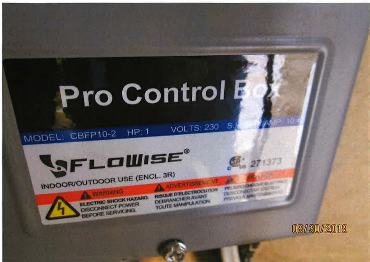
1 HP pump in well. Theoretical pumping equation estimates the flow rate at 0.04 cfs.
