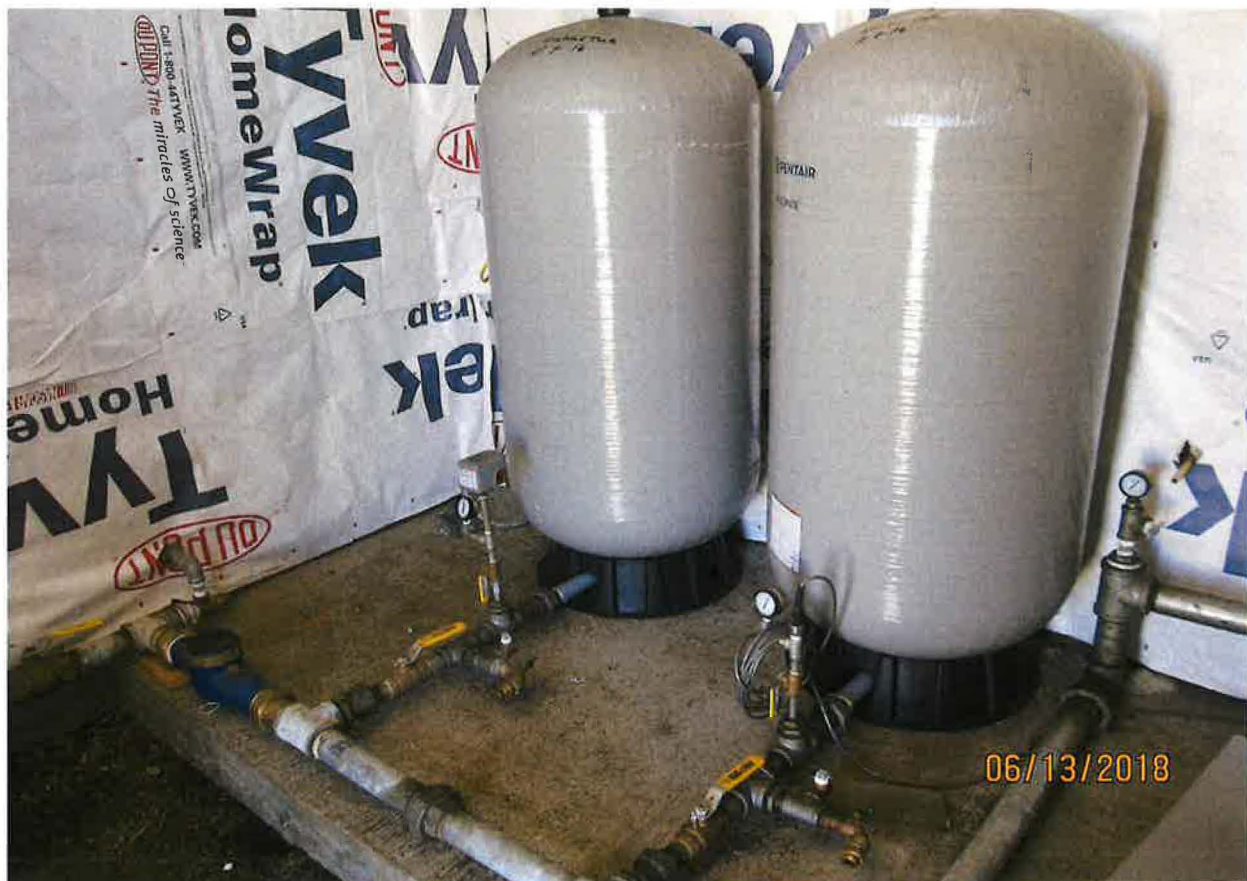
Water from storage tank to pressure tanks to homes
