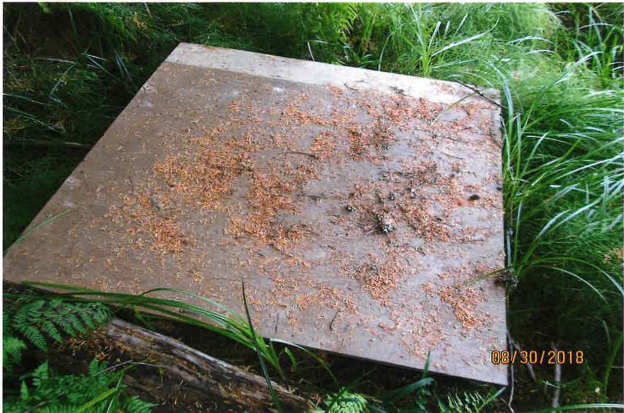
POD – SPRING BOX WITH SUBMERSIBLE PUMP
