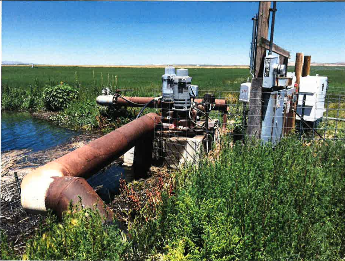
Holding pond where ground water is pumped to. Water in small pond is collected from other sources and enters booster system to pivots and sprinklers.
