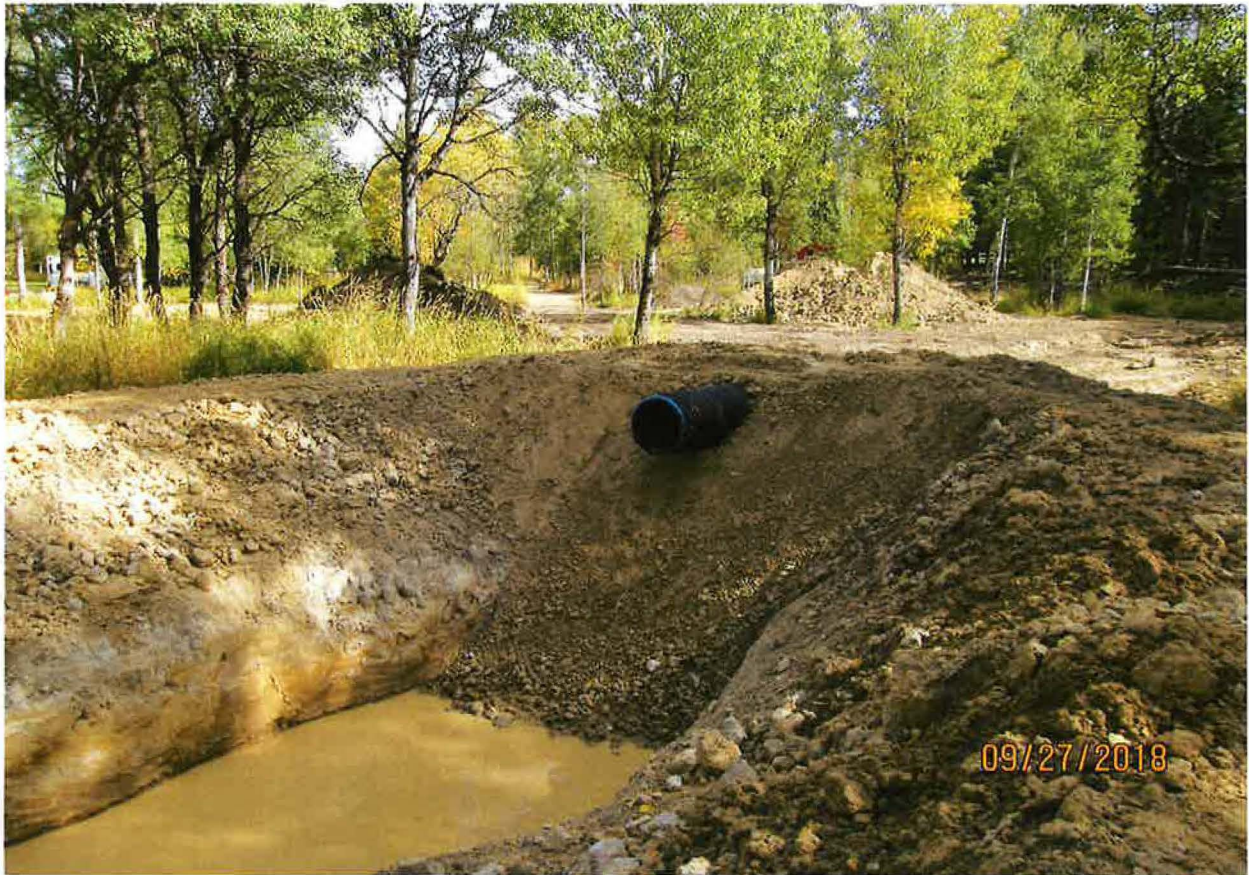
POND OUTFLOW CULVERT
