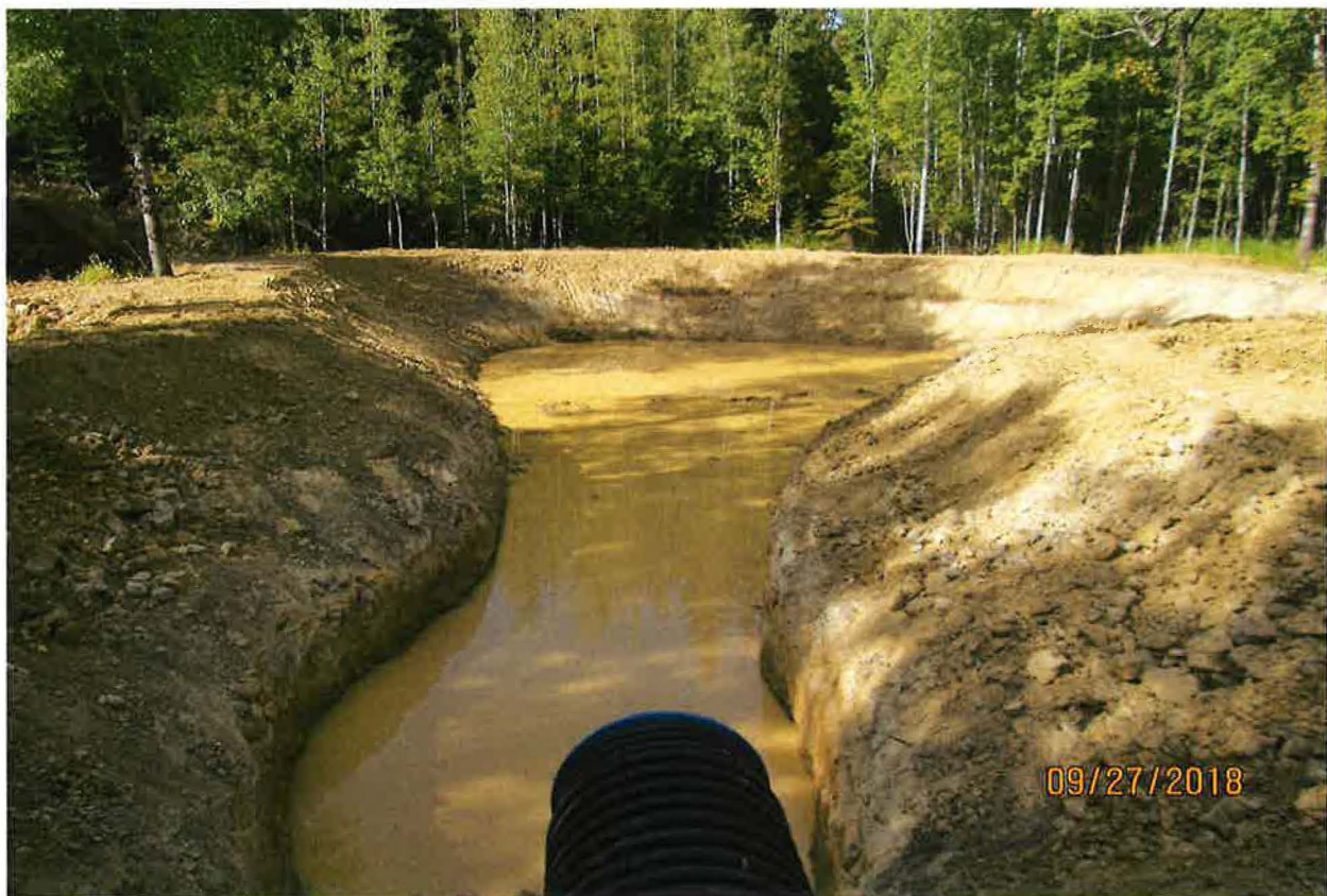
POND OUTFLOW CULVERT
