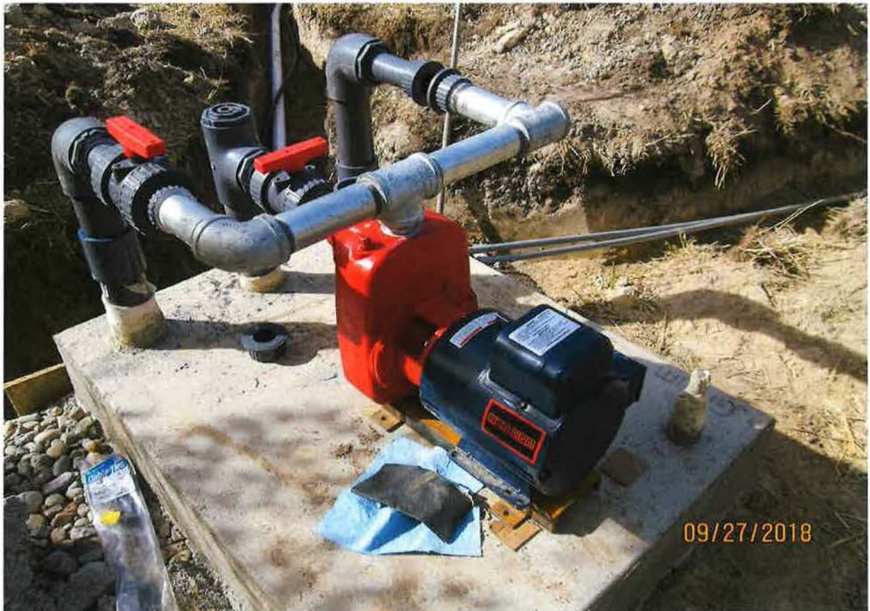
3 HP PUMP FOR IRRIGATION FROM STORAGE
