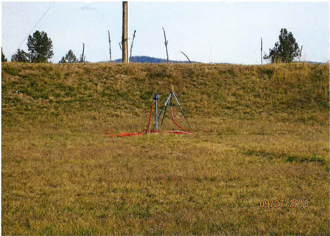
IRRIGATION POU – FROST FREE HYDRANT AND HOSE FED SPRINKLER
