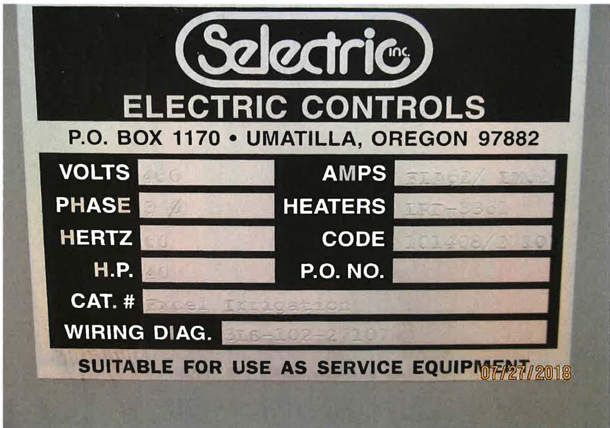
Pump tag showing 40hp pump.
