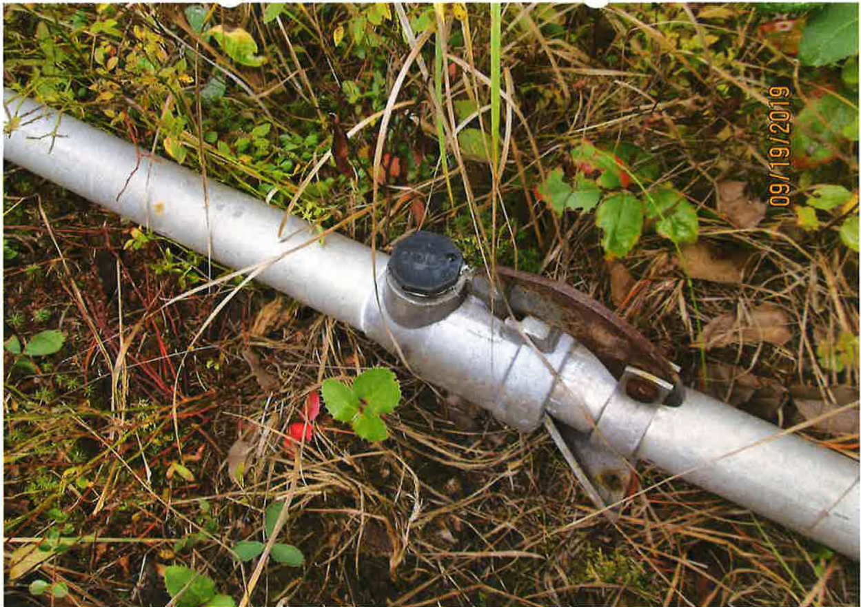
POU SPRINKLER PIPE / PRESSURE GAGE INSTALLED HERE TO DETERMINE OPERATING PSI
